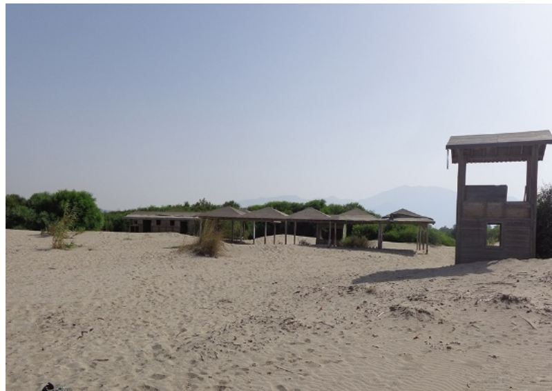
Letoon beach: the former SPA facilities that are not in use, remain on the beach in a state of decay.
