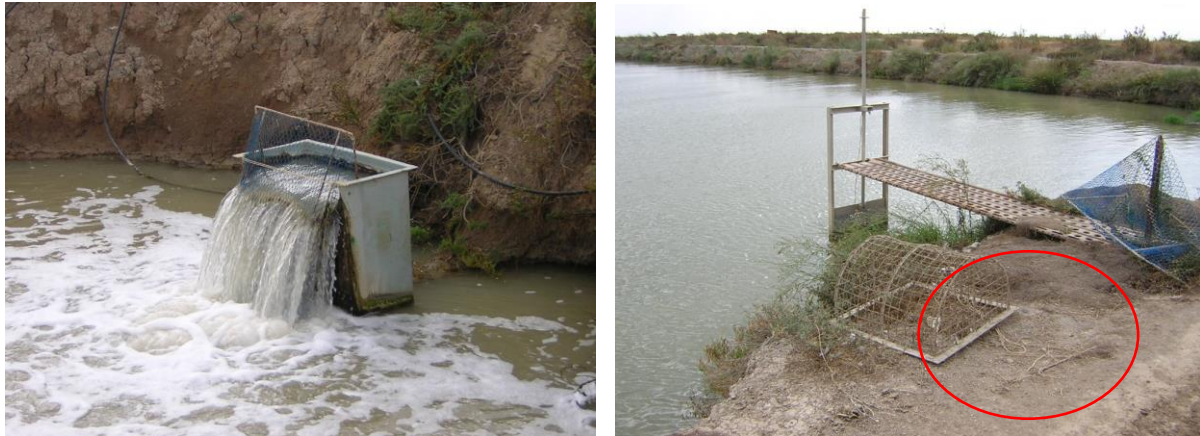
Figure 5.11: Inflow of a semi-extensive pond equipped with a spherical filtering screen (red circle) mounted (left) and detached (right). (Photo credit: M. Chebanov).
