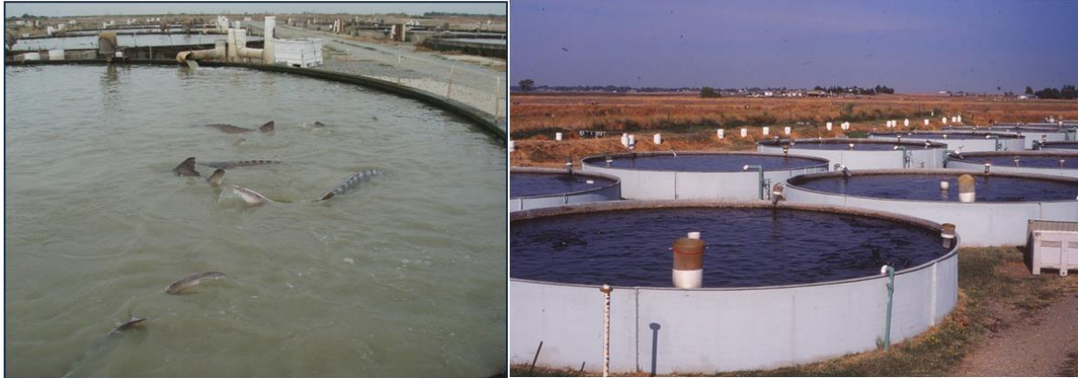
Figure 5.5: Concrete (left) 15 m diameter, and fiberglass (right) 6 m diameter circular tanks used for A. transmontanus broodstock rearing (Photo credit: J.P. Van Eenennaam).
