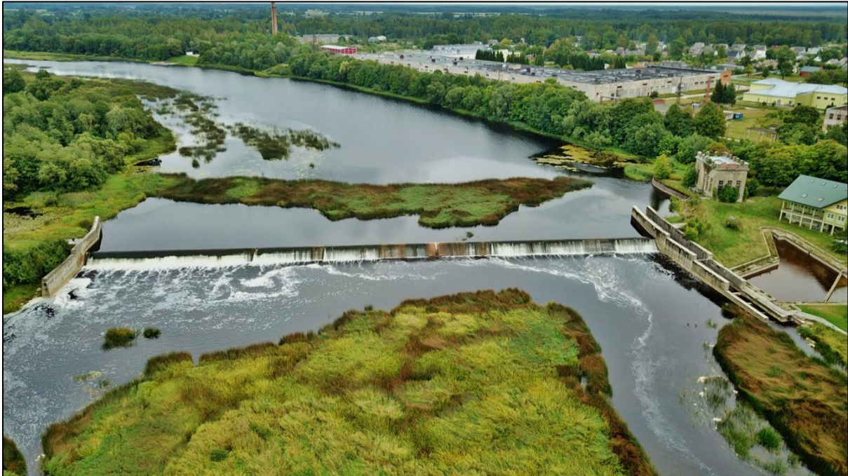
Figure 4: Sindi dam on the Pärnu River in Estonia. Migration barrier for sturgeon and other fish. Note the fish pass on right side of photo (© Jarko Jaadla).
