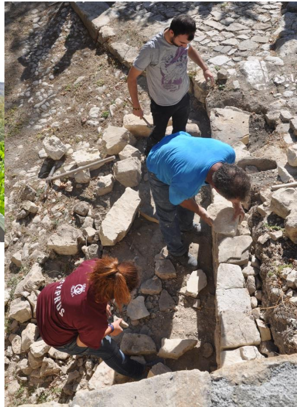
✓ Dry masonry workshop
