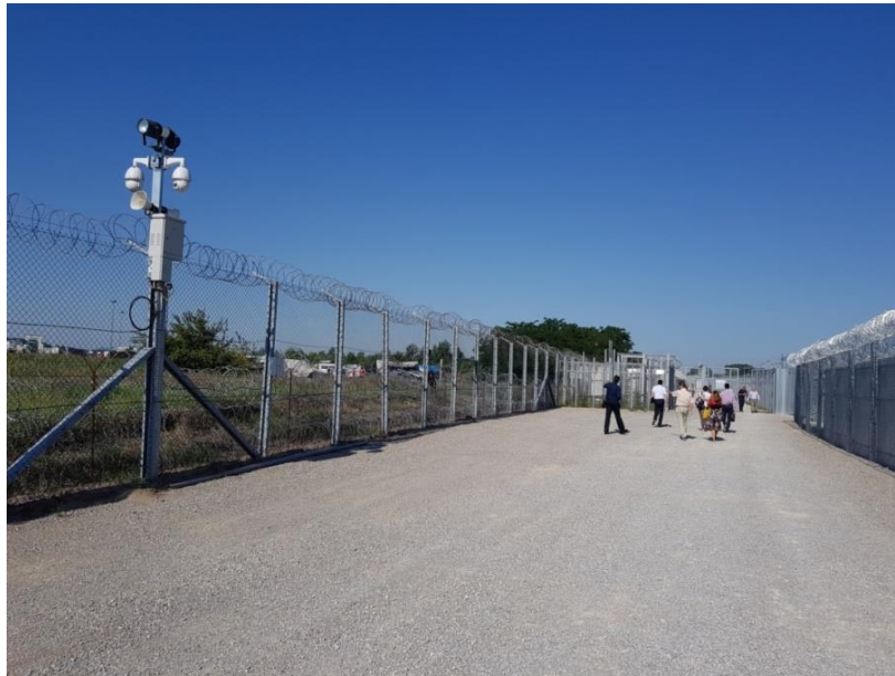
(Entrance of Rösztke transit zone for visitors and employees, from the Hungarian side)
