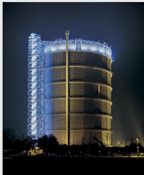
■ Built between 1927–1929 to store gas for smelting and coking processes, and with a storage capacity of 350,000 m<sup>3</sup>, the Oberhausen Gasometer is the largest disc-type gasometer in Europe. Following the closure of the neighbouring industrial plants in 1988, the gasometer became superfluous and was seen by the public as an oversized symbol of the industrial decline of the region.
