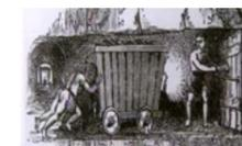
To clear coal mines of gas a crude system of ventilation was used. To assist this, young children called trappers would sit underground opening and shutting trap doors which went across a mine. This allowed coal trucks through but it also created a draught and it could shift a cloud of gas. However, it was very ineffectual. It was also believed that a system of trap doors might help to stop the blast of an explosion damaging more of the coal mine.
