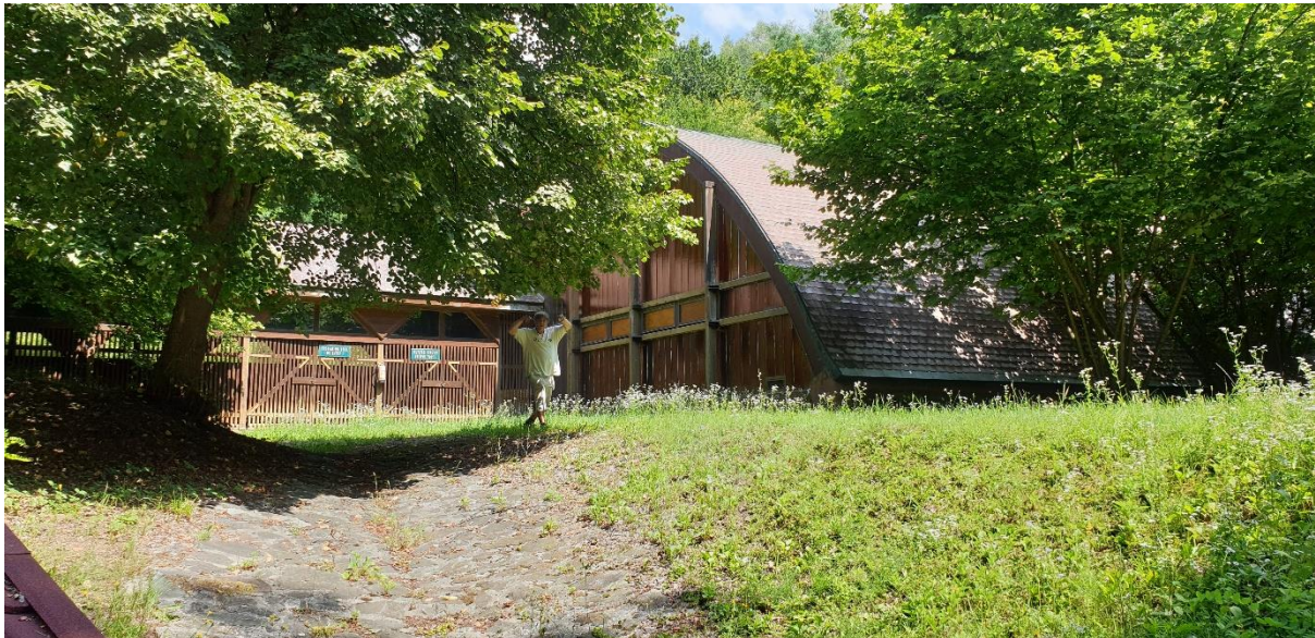
The Grand Hall, one of the exhibition buildings along the Geological Study Path.
