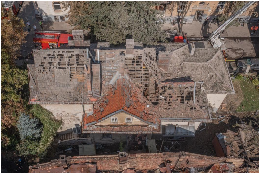
Figure 1. Damage to the “Sunny Villa” in Lviv following a missile strike on 4 September 2023. The building is located within the UNESCO-listed historic centre and its buffer zone, which sustained damage to multiple heritage sites during the attack.
