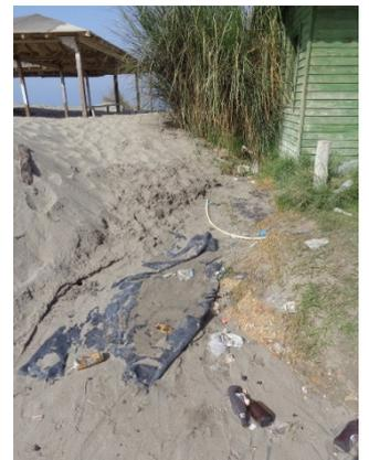
**Figure 8: wet sand around leaking pipe and tube**
