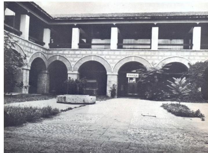
after reconstruction (RC elements)
