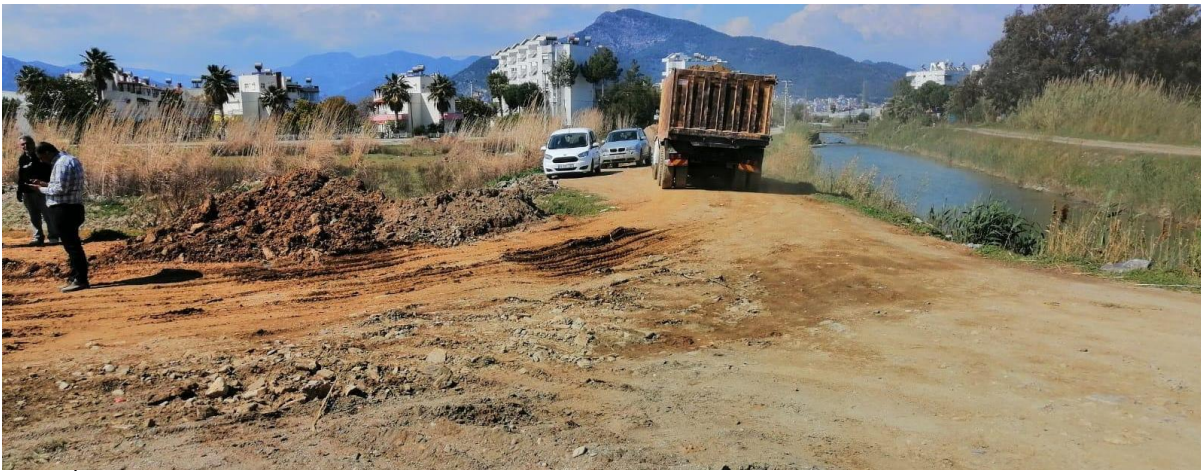
Fig. 2 | Karaağaç 31 March 2021: Heavy machinery removing illegally placed soil for picnic area.
