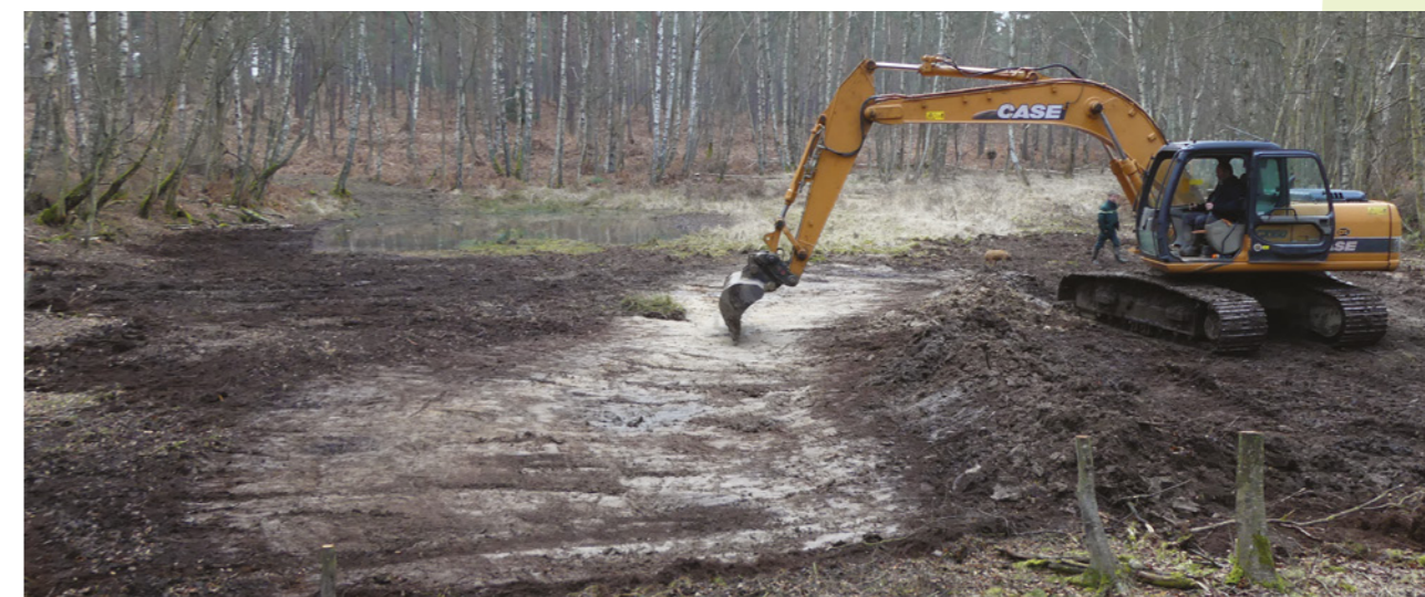
Topsoil and vegetation removal to restore rich acidic forest ponds in Rambouillet forest, France - A. Potier CBNBP/MNHN
