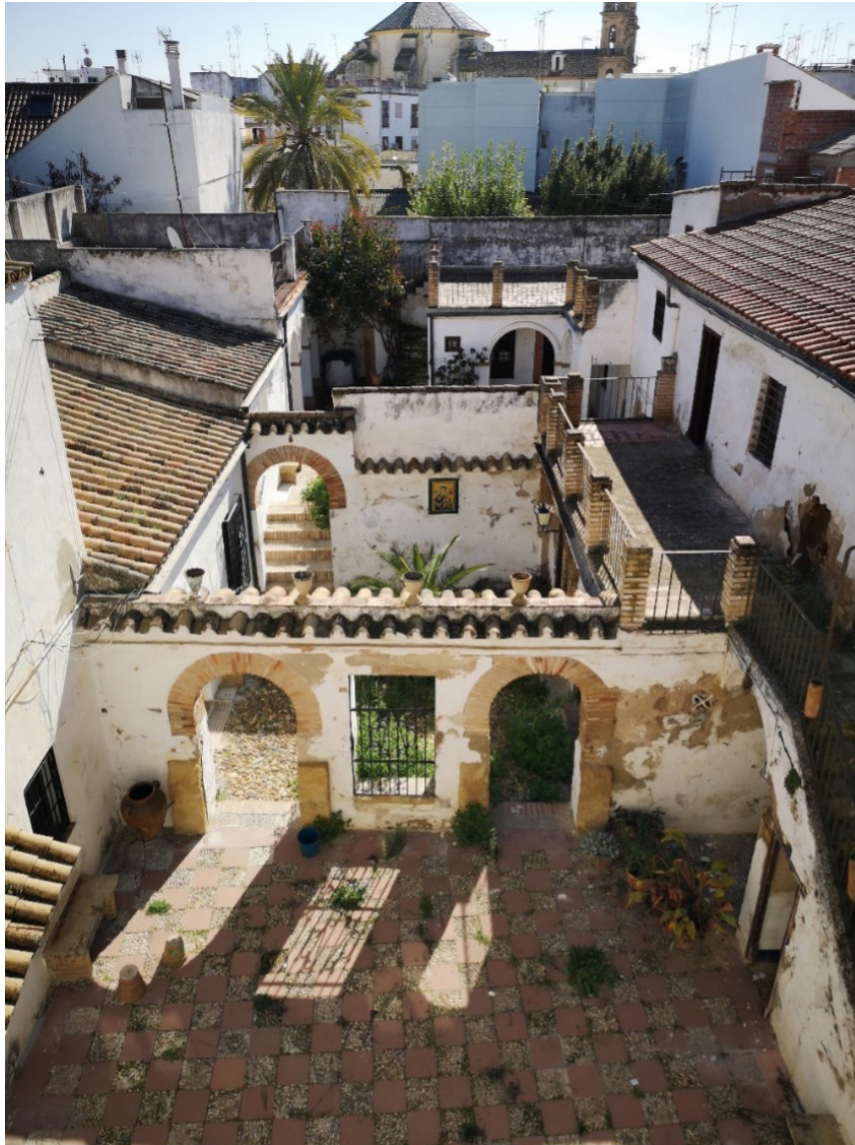
Image of the PAX Astronauts House before the construction. Photo: Gaia Redaelli
