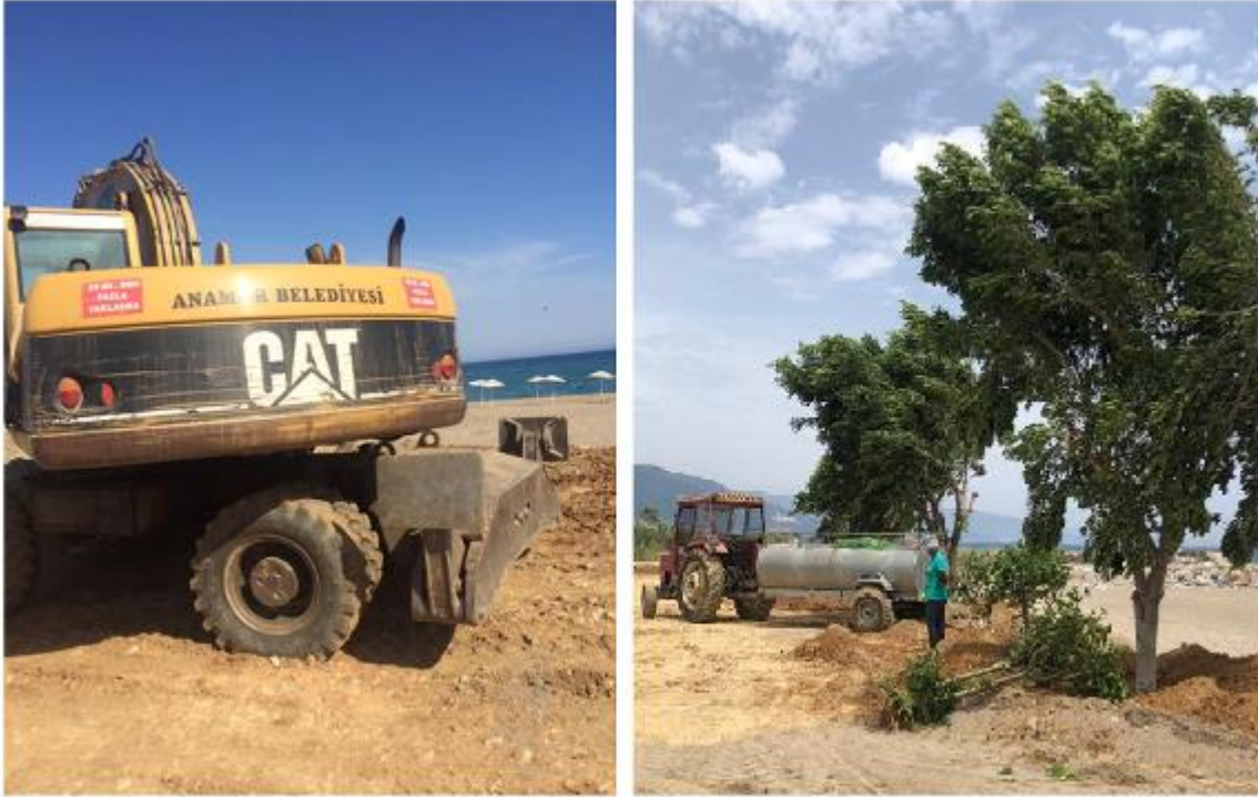
Figure 8 - Heavy machines working at the beach
