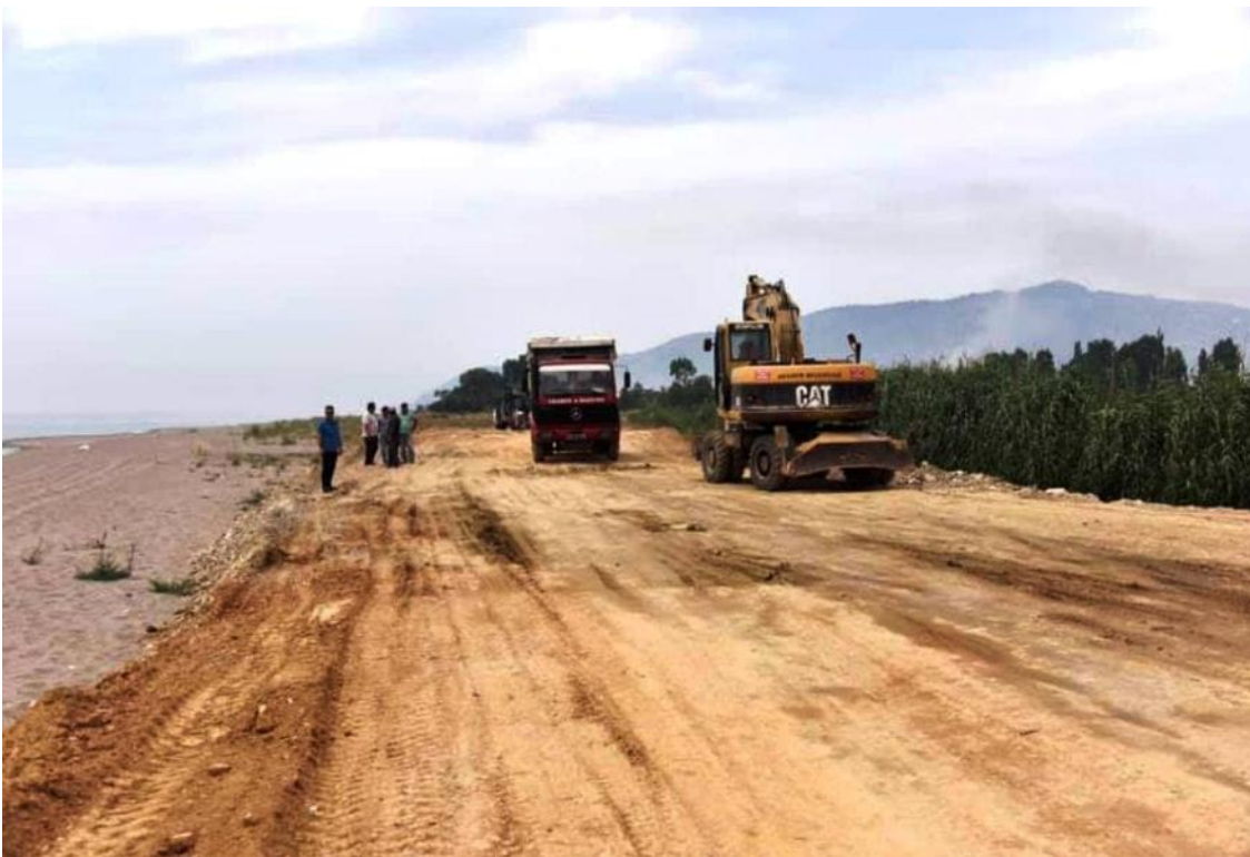
Figure 9 - Soil laid on the beach
