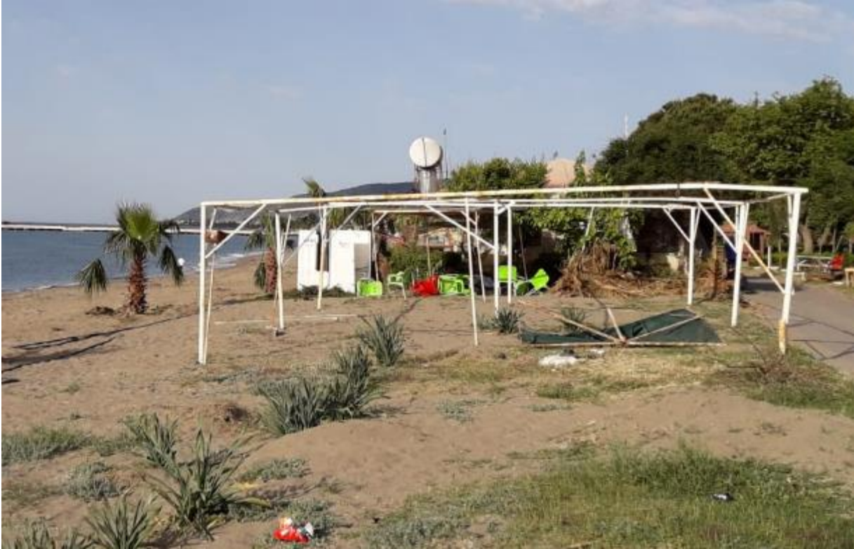
Figure 47 - Illegal Construction on the Beach
