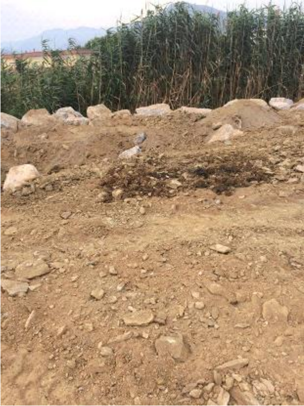
Figure 20 - Stone Wall Built inside the Creek
