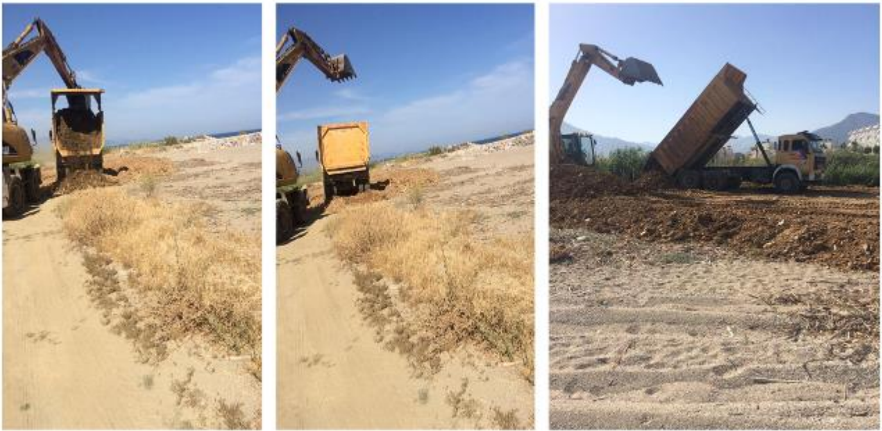
Figure 6 - Machines Poured Soil on the Beach (First Day of Construction-31.05.2019)
