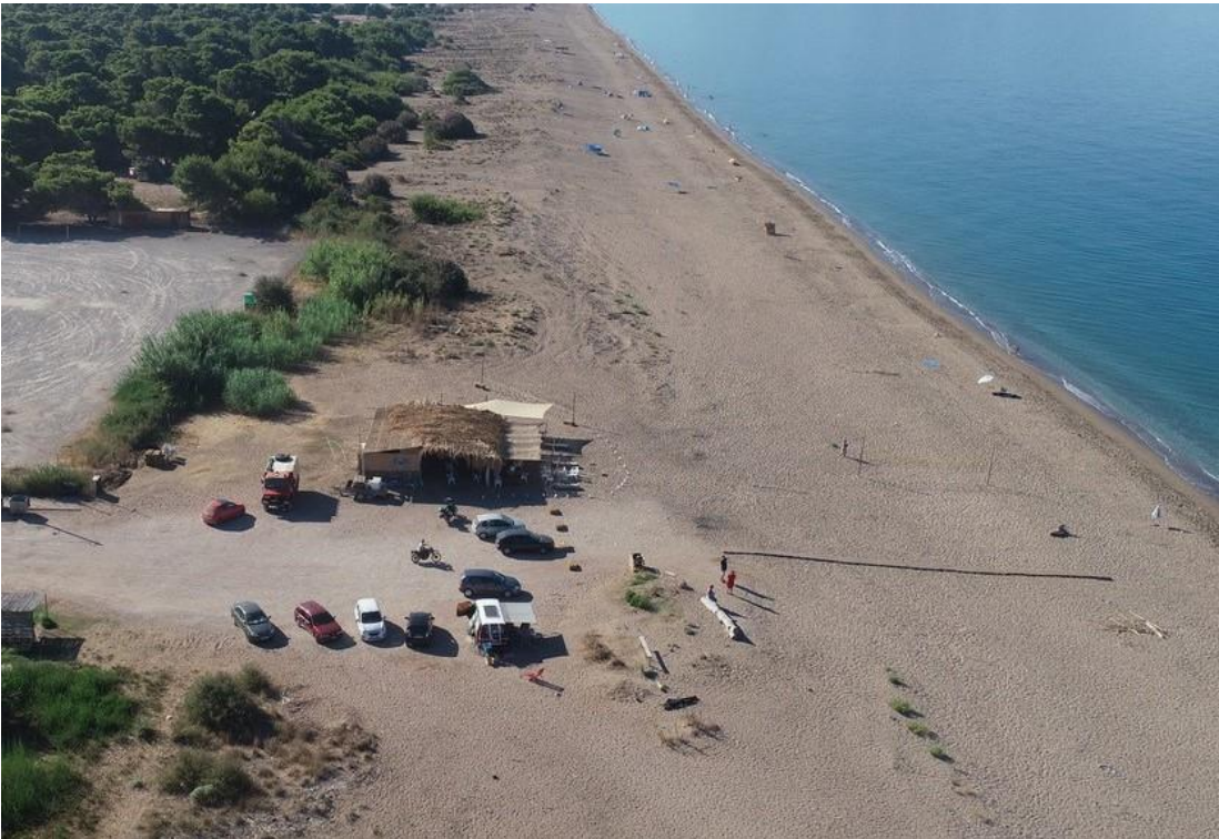
Photo 5: The beach bar at C sector (Elaia) operated on the dune zone and caused further deterioration of the habitat.
