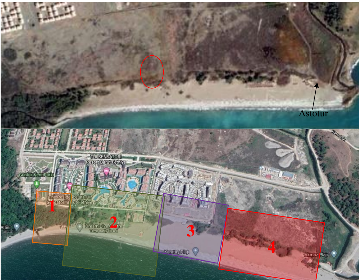
Fig. 4. Fethiye SPA, Karataş. Google Earth images from 2003 (top) and 2020 (bottom). From left to right in the 2020 image: 1) Günlük Kent Park, 2) TUI Sensatori Resort Barut and its residence section, 3) ongoing new construction site (Fabay Koymat Hotel), and 4) the project sites for two new hotels (Three Sisters-1 – Lillyana Resort and Three Sisters-2 – Aronis Resort). The once pristine nesting beach is now covered with pavilions and sunbeds at the western end, although sunbeds seem to be placed behind the nesting zone towards the east of TUI Sensatori.
