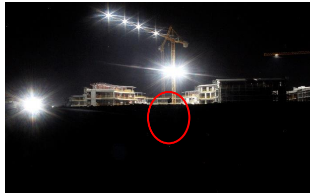
Fig. 24b. Fethiye SPA, Karataş. Construction lights on the nesting beach. Note the cage in front of it.
