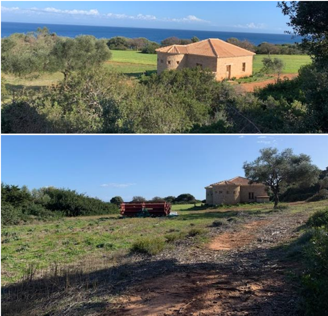
Fig. 1-2. Illegal Building in Gerakas, 31.01.2021
