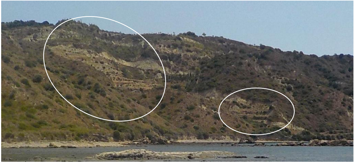
Fig. 10 | Illegal Road between Gerakas and Daphne, Pre & Post Google Earth Images (top), Photo taken 14 th July 2021 (bottom). No signs of restoration work carried out to return the protected area to its natural state; the road carved into the protected landscape is still clearly visible in the photo (white circles).
