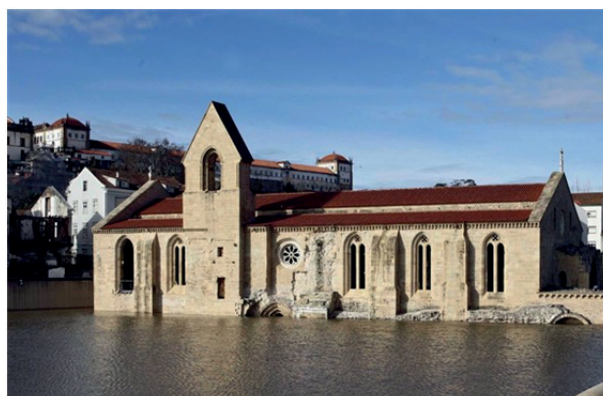
1. - Monastery of Santa Clara-a-Velha in Coimbra, Mondego river floods 2016. Accessed July 25, 2017, http://www.dn.pt/sociedade/interior/mosteiro-de-santa-clara-encerrado-ate-domingo-4978620.html .
