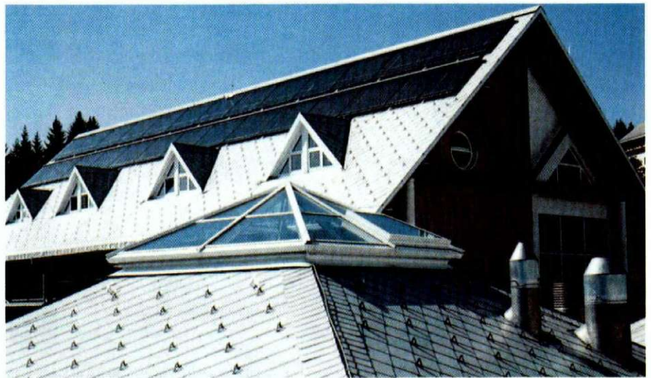
A very interesting example of solar heating facilities: "Haus Gertrud"
