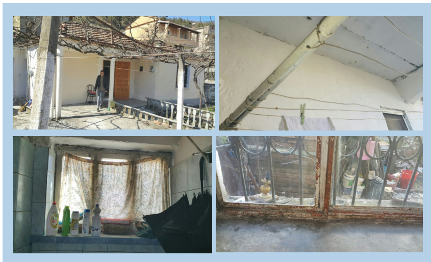
Figure 4. Field observation on needs assessment in the Housing area
