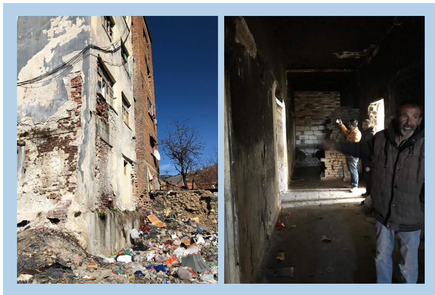
Figure 2. Pictures from field visits (former dormitories)
