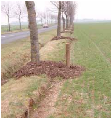
III. 106: Posts used to protect trees from damage in France. If the trees had been planted on the verge, between the roadway and the ditch, the risk of impact damage would have been minimised while at the same time restricting root growth in the direction of the cultivated land. III. 107: A strip of fallow land – here in Sweden – provides protection against impacts and soil compression
