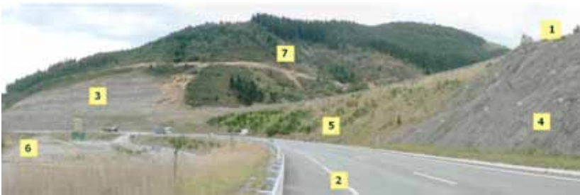
Ill. 76: Construction of a separated dual carriageway to expand capacity. Earthworks, particularly those of high-speed and high-capacity roads, determine road presence in the landscape. Road infrastructure involves a variety of elements, such as separate lanes (1 and 2), embankments (4 and 5), cuttings (3), service side road (7), and building installation areas (6)
