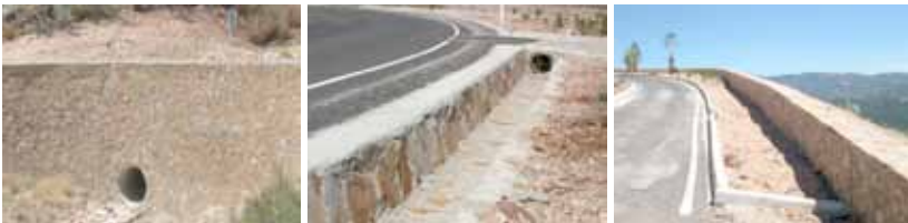
Ills. 60, 61 and 62: Sandstone is a consistent material which, when used in different roadside elements (retaining wall, drains and parapets), builds up a sense of identity
