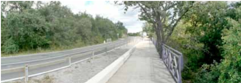
III. 50: Separate bicycle lane. Safety barrier and low parapet separate pedestrians from traffic
