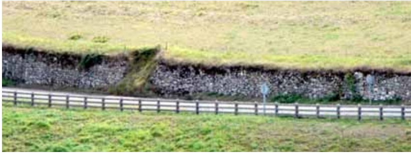
III. 25: A traditional stone wall works as a retaining wall for the road cutting, while the embankment has been successfully laid to grass so as to give it a natural feel
