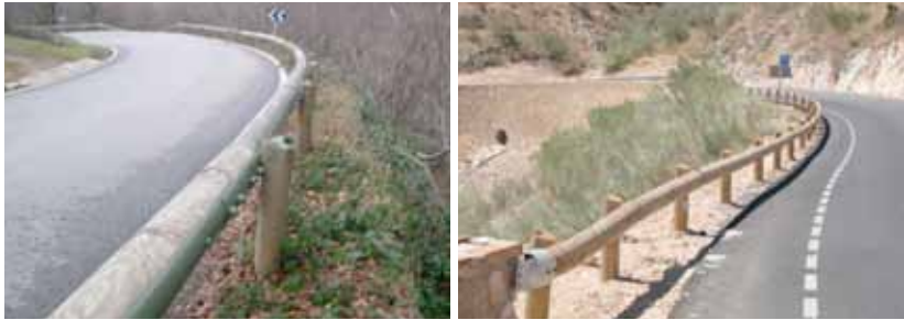
Ills. 18 and 19: Wooden safety barriers on roads provide a sense of the natural and rural. However, as increasingly used standard elements, they run the risk of creating a lack of identity
