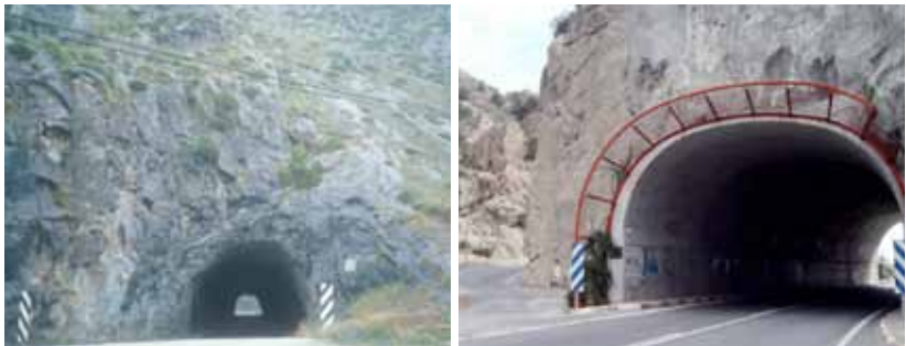
Ills. 41 and 42: Mouths of two tunnels. (Left) Carved tunnel for a one-lane road on the island of El Hierro (Spain). (Right) Red ornamental protection marquee and plastered rocks at a tunnel in the Ricote Valley, Murcia (Spain) (photo by L. Cruz)
