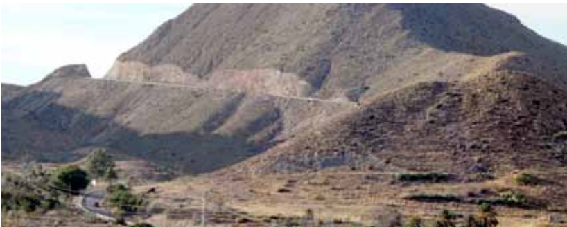
Ill. 77: Slope cutting of roads produces a “scar effect” on the landscape, which can only be partially reversed when the slope allows through revegetation measures and rock treatments
