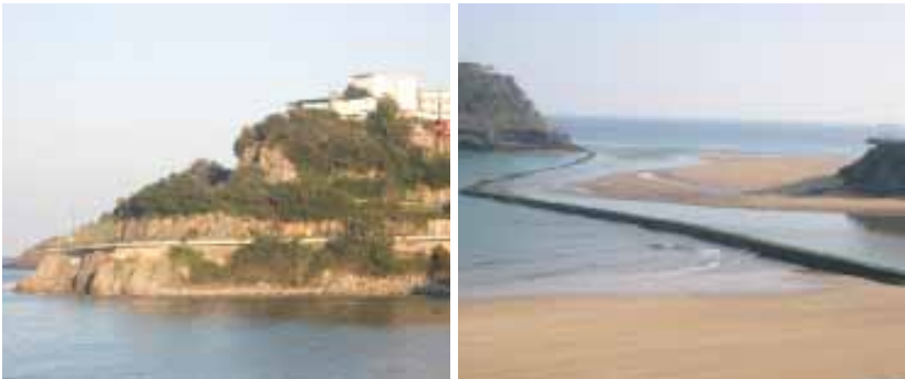
Ills. IV-4 and IV-5: (Left) The Karraspio road cuts into the rocky slope. The cuttings of the main road to Ondarroa are noticeable above. Note the flying platform on the left. Sea is at high tide. (Right) The dam for the tide mill shows its alignment from Saint Nikolas Island to the river mouth at low tide. Note, on the right of the picture, the flying platform of the road to Karraspio
