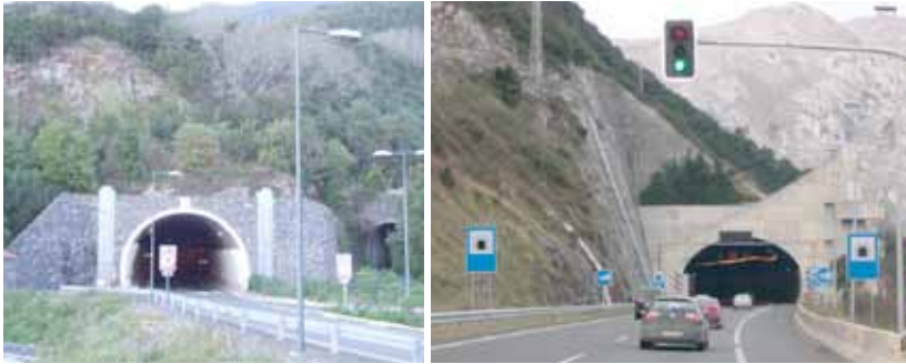
Ills. 43 and 44: Mouths of two more tunnels. (Left) Structure covered by stone wall on the island of La Palma (Spain) (photo by J.T. Rodríguez). (Right) Sophisticated ornamental walls for the Cantábrico Motorway (Spain). Note in both cases the slope of the hillside above the tunnel is partially integrated into the external design
