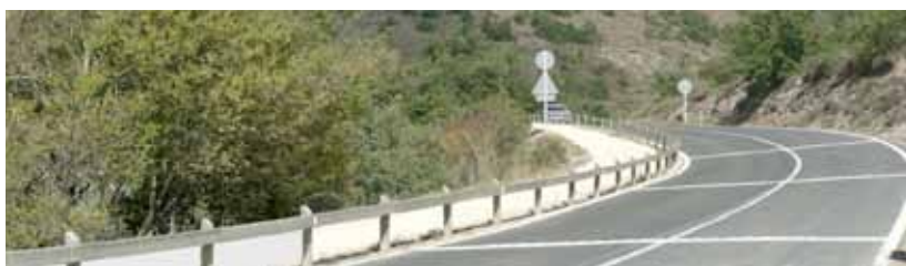
III. III-11: Speed reduction marks on the road and a low safety barrier create more footpath safety and comfort
