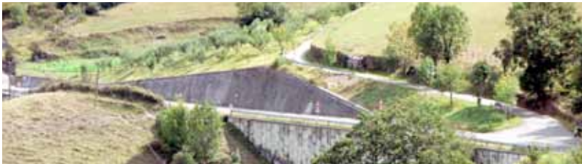
Ill. 24: The picture above shows a road the embankment of which is supported by a prefabricated slabbed wall partially hidden behind a tree on the right side of the picture. The road cutting on the same stretch leans on an inclined concrete retaining wall, which helps to support both the slope and a ramp
