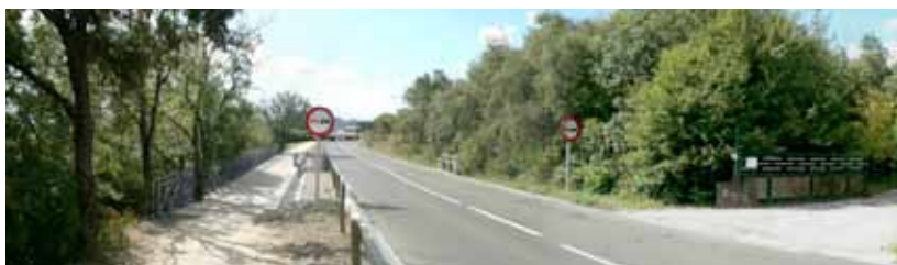
III. III-10: The side platform (on the left) respects vegetation on both sides of the road, encouraging ecological connectivity
