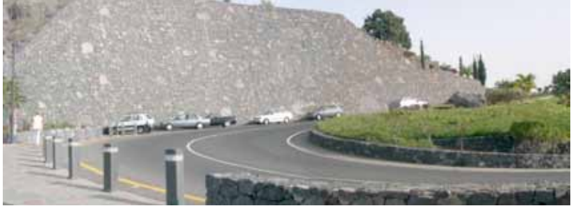
Ill. 63: The parapet in the foreground is a traditional stone wall that is integrated with modern materials, such as the safety bollards. In the background a retaining wall is covered with traditional black stone, while at either end there are local plants and trees and large rocks as well. All these elements together manage to create a sense of identity for the road
