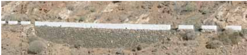
III. 26: The road platform is held by a retaining wall concealed under a finish of traditional stone walling. Traditional stone walling and an old-fashioned white parapet provide a good result in functional and landscape terms
