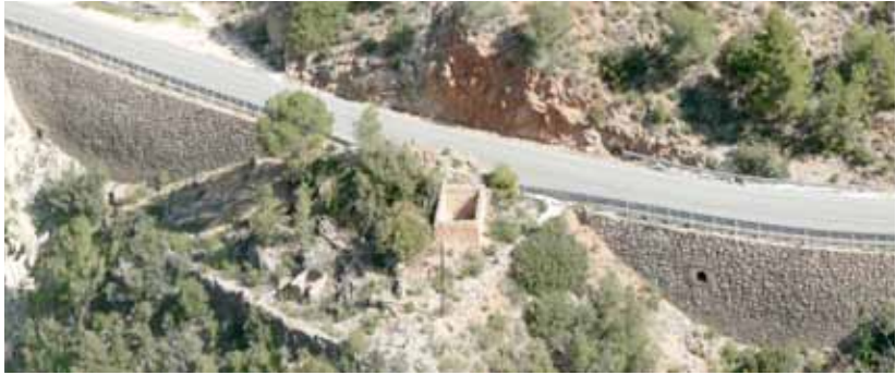
III. 78: Stone walls as retaining walls have a positive effect on landscape
