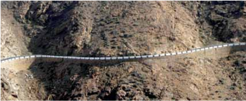
III. 80: Traditional character elements, such as a teeth-like safety barrier and retaining walls made from local stone, encourage positive landscape integration
