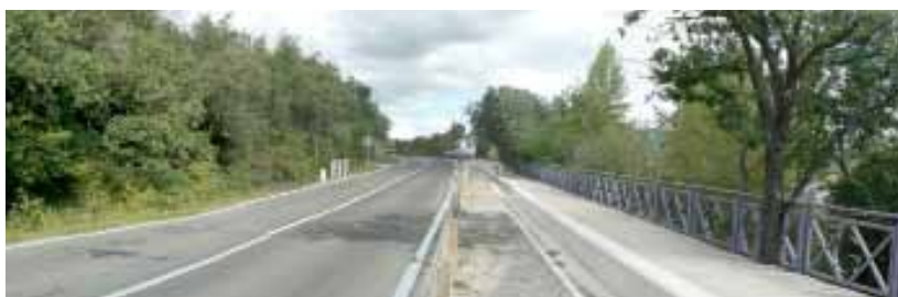
III. III-8: Construction of a side platform has enabled a footpath to be built adjacent to the A-3002. A white parapet and a safety barrier separate pedestrians from traffic and a guardrail prevents access to the shore
