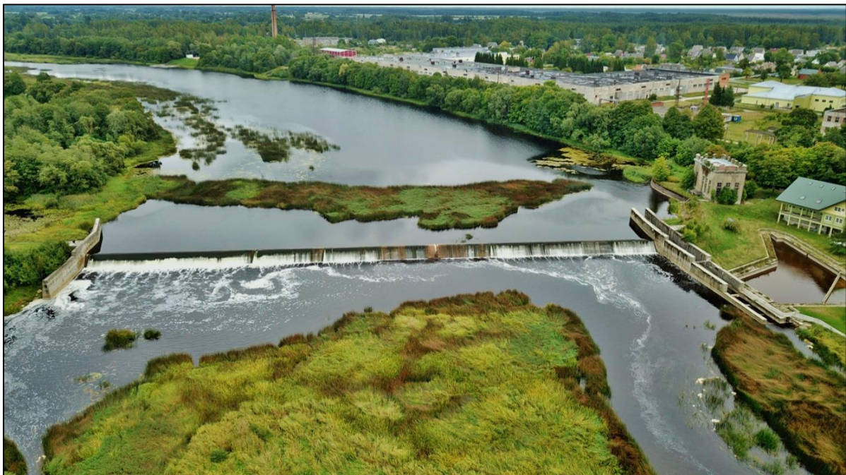
Figure 4: Sindi dam on the Pärnu River in Estonia. Migration barrier for sturgeon and other fish. Note the fish pass on right side of photo (© Jarko Jaadla).
