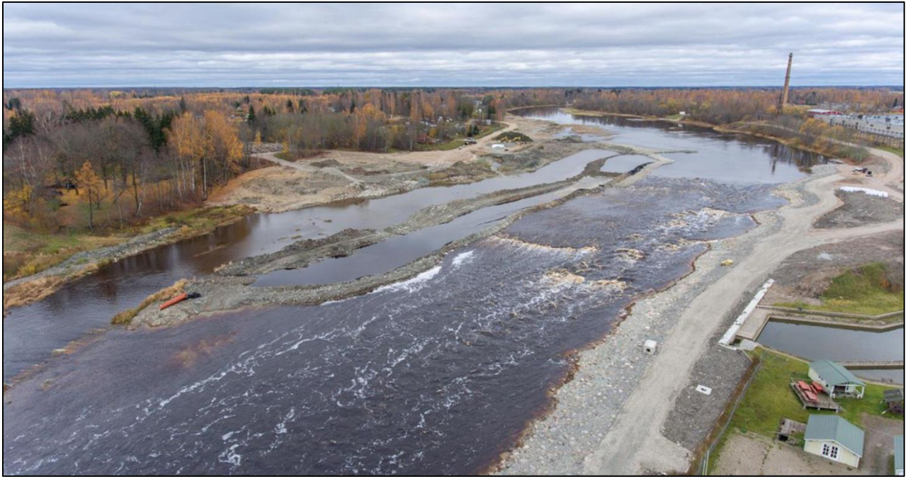
Figure 5: Pärnu River in Estonia after removal of the Sindi dam. River continuity for migratory fish has been restored (© Keskkonnaamet).
