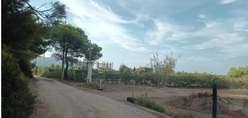
Photos 6c, 6d: Location Vounaki (A Sector) – September & October 2024 – Construction of 2 new houses within the NPZ-2c.
