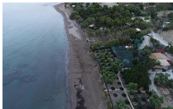
Photo 4: Illegal constructions and businesses on Daphni beach.
