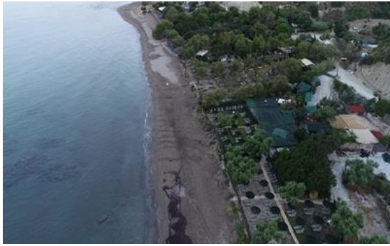
Photo 4: Illegal constructions and businesses on Daphni beach.
