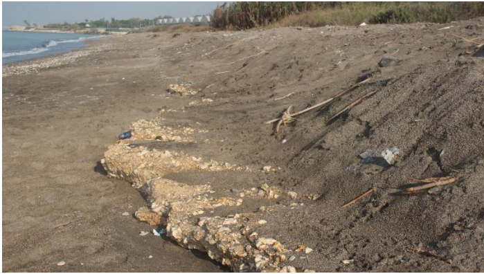
Fig. 5. Kazanlı. Section K3. July 2021. Exposed stone and cement mixture under the sand.
