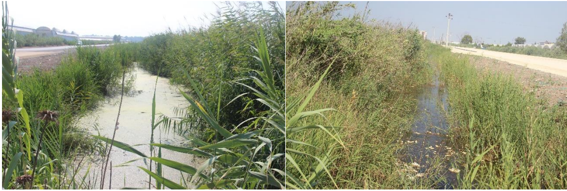
Fig. 47. Kazanlı. July 2021. Polluted drainage channels adjacent to the main road behind K2 and K1
