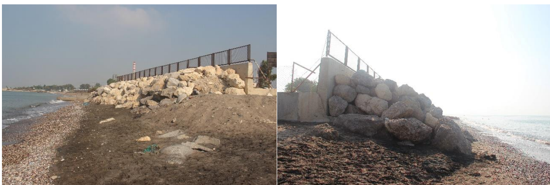
Fig. 33. Kazanlı. Section K2. July 2021. Arbitrary use of boulders in front of the local schoolyard.
