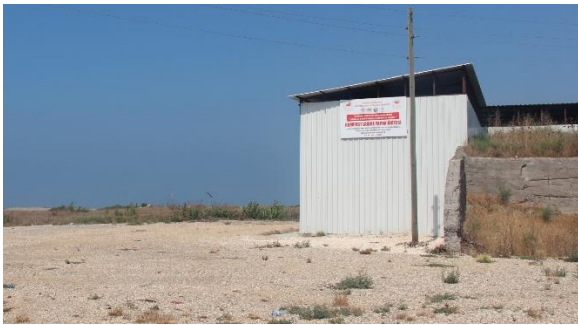
Fig. 48. Kazanlı, Section K1. July 2021. Composted fertilizer production unit at the back of the beach.
