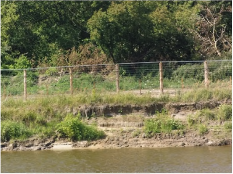
Photo 17. A fence built along the river.
