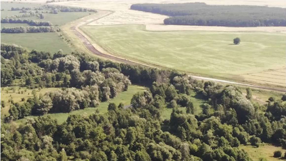
Photo 18. The fence is built along the flood embankment, near Włodawa.
