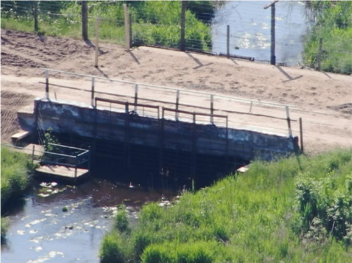
Photo 15. A tight dam on the river, near Włodawa.
