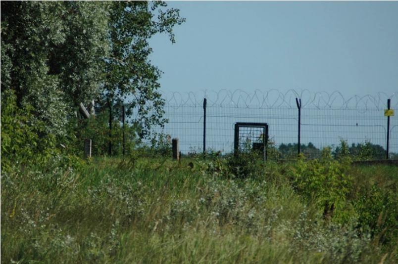
Photo 11. Wicket in the modernized fence used by border services, near Włodawa.
