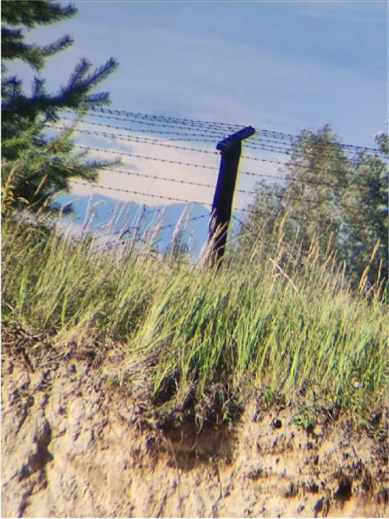
Photo 16. A fence built along the river.
