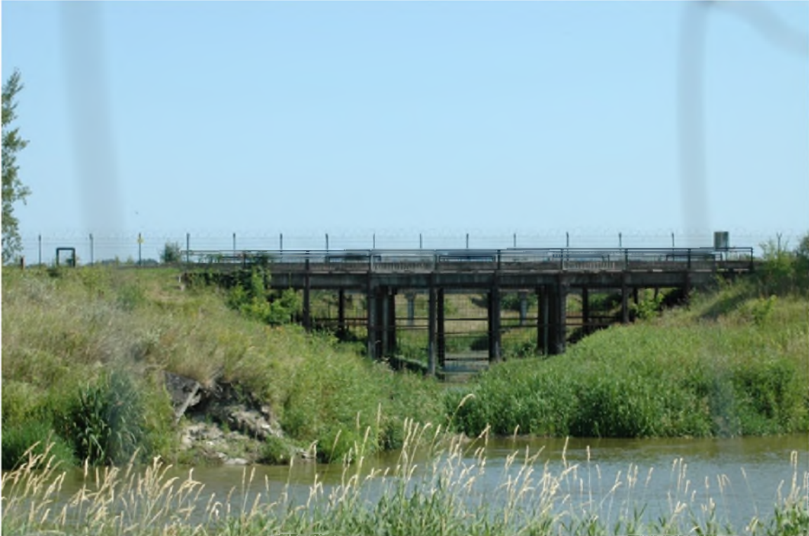
Photo 14. A tight dam on the river, near Włodawa.
