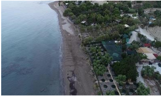
Photo 4: Illegal constructions and businesses on Daphni beach.
