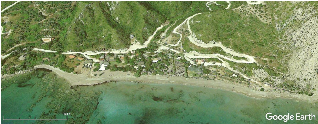
Fig. 3 | Daphne; 2020 Google Earth image: Natural sand dune system destroyed. All the buildings seen in this figure are illegal.
