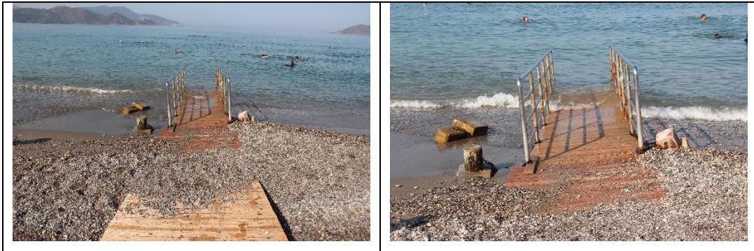
Fig.7. Fethiye SPA, Çalış B. Scaffold for the impaired, fixed by chains, large stones and cement. Note the walkway extending all the way to its back (7a).
