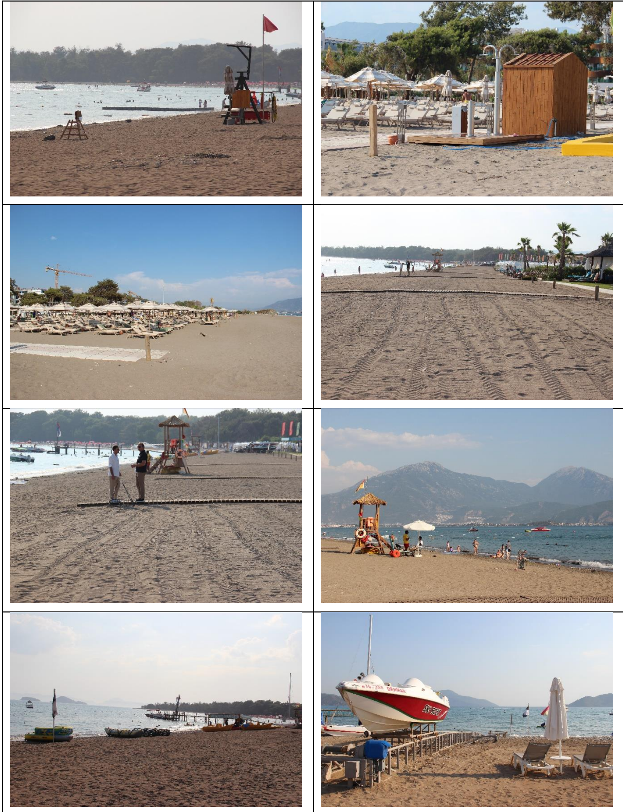
Fig.25. Fethiye SPA, Yanıklar. Enlarged beach of Liberty Fabay. a) A new lifeguard tower, custom-made prism cage, and jet-skis in the sea; b) new sunbeds, umbrellas, and a showering space draining onto the beach; c) general view of enlarged area, another lifeguard tower, and replaced zoning stakes; d-e) vertical walkways, sand flattening tracks, an old prism cage and jet-skis in the sea -note the artificial plantations in (d); f) the new lifeguard tower and jet-skis in the sea; g-h) water sports equipment.
