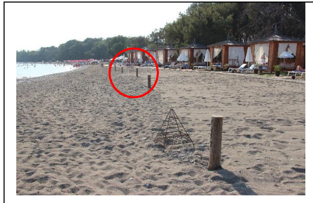
Fig.27. Fethiye SPA, Yanıklar. Zoning stakes in front of TUI's pavilion area, incorrect zoning.
