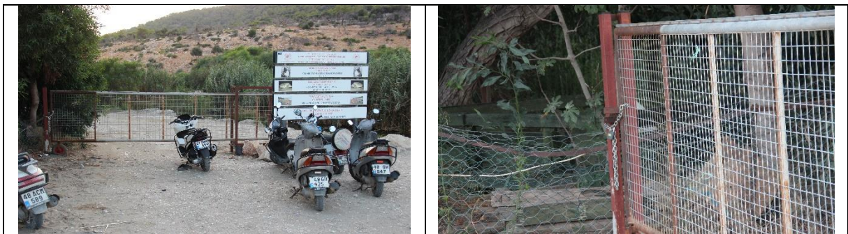
Fig.33. Patara SPA, Özden Beach. Chained and locked barrier at the beach entrance point. Note the old Ministry warning sign (a).
