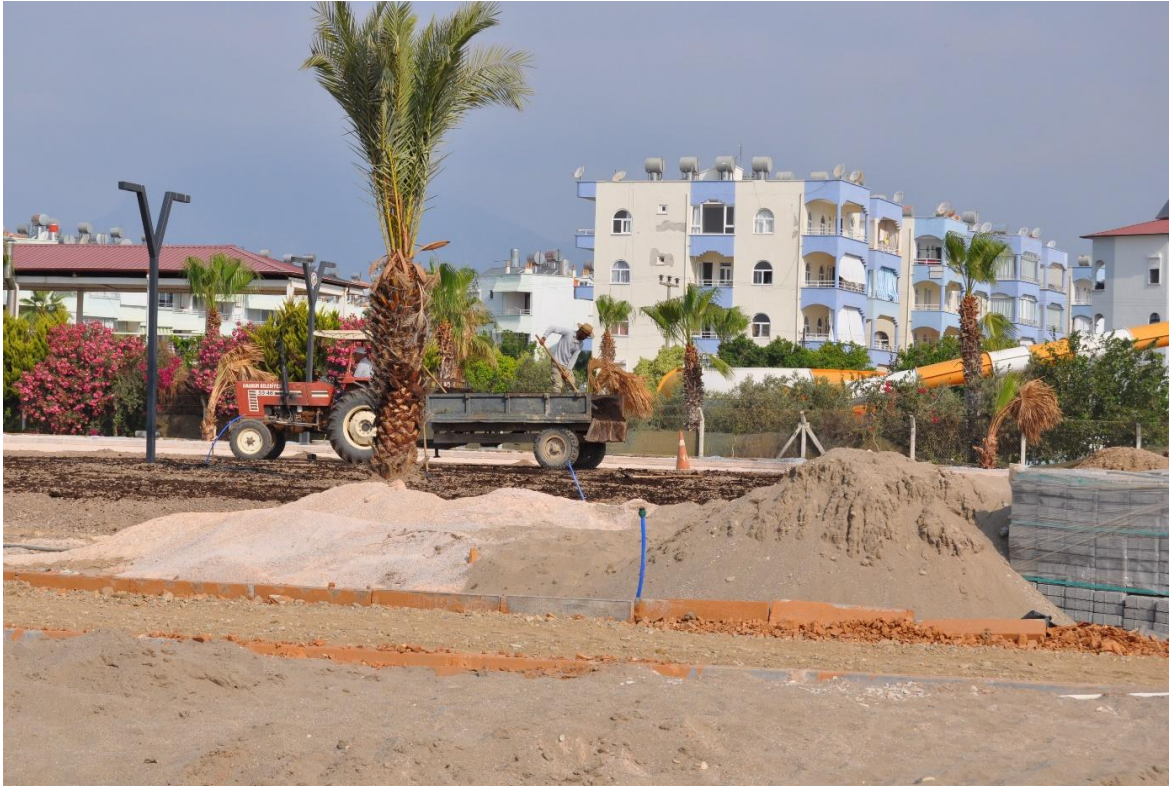
c) Soil brought to the field for filling and use of fertilizers for germination on backwards July 2023
