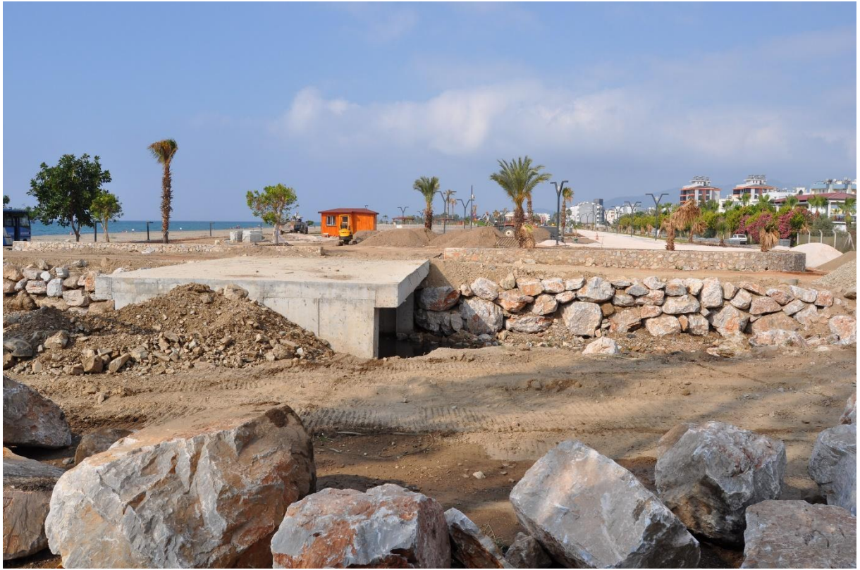
a) Construction activities within the secondary protection zone continue - July 2023
