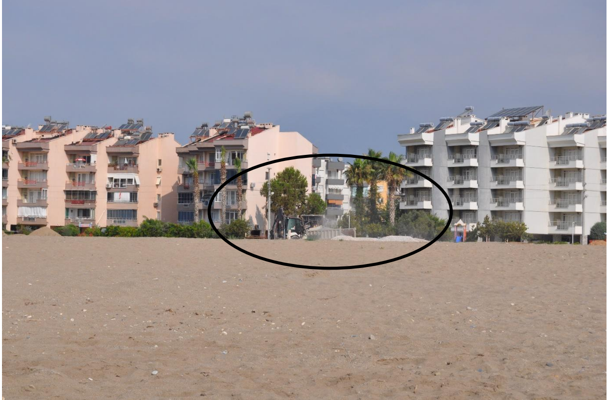
e) Project construction activities are still continuing despite the 2009/10 circular - July 2023
