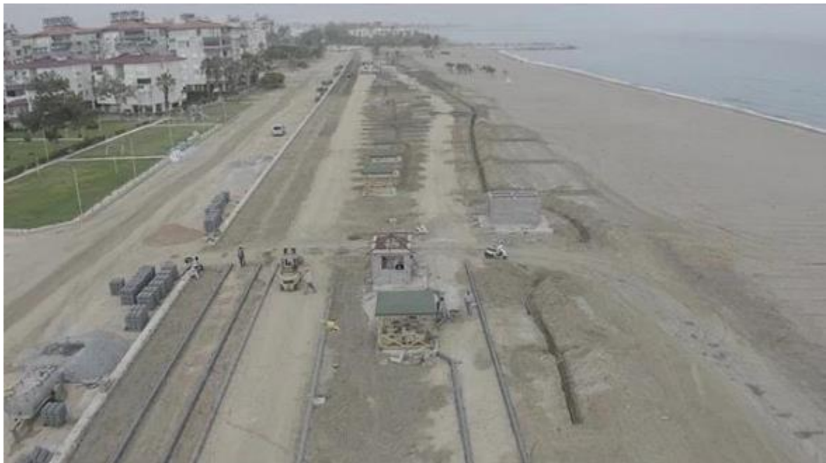
f) Beach Arrangement Project construction - Phase I - November 2021
