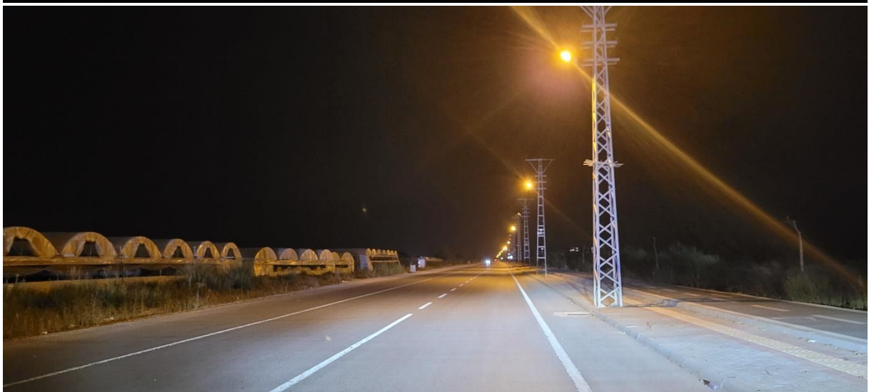
Fig 10. Road lights are amber and they are not visible from the beach.
