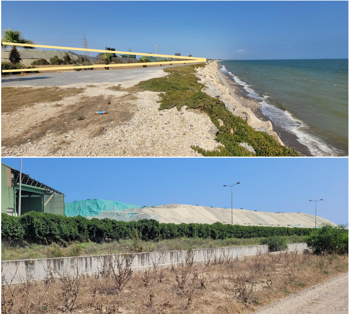
Fig 20. The chemical waste storage areas maintained their current location and condition
