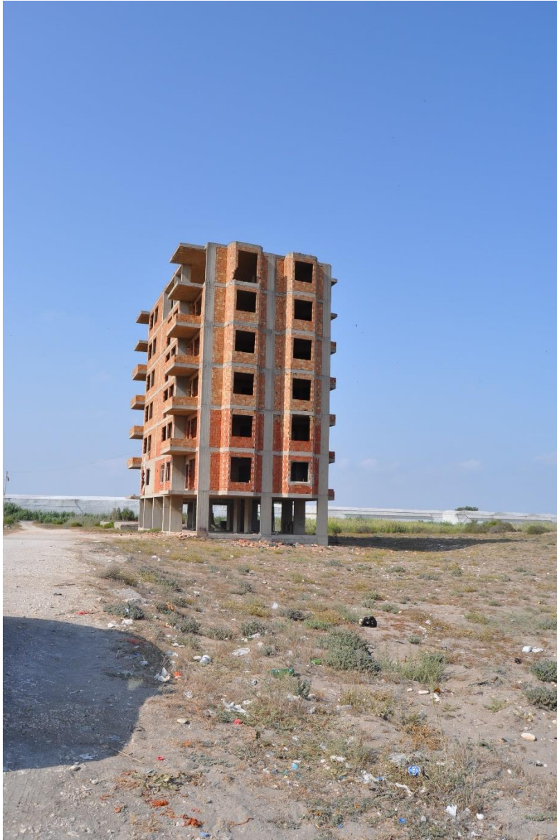
Fig 19. The illegal building is completely abandoned
