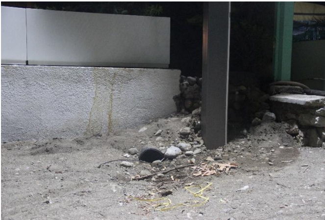
Fig.58. Fethiye SPA, Yanıklar. Plastic drainage pipe outlet at the base of security light's post between Okaliptüs and Tuana.
