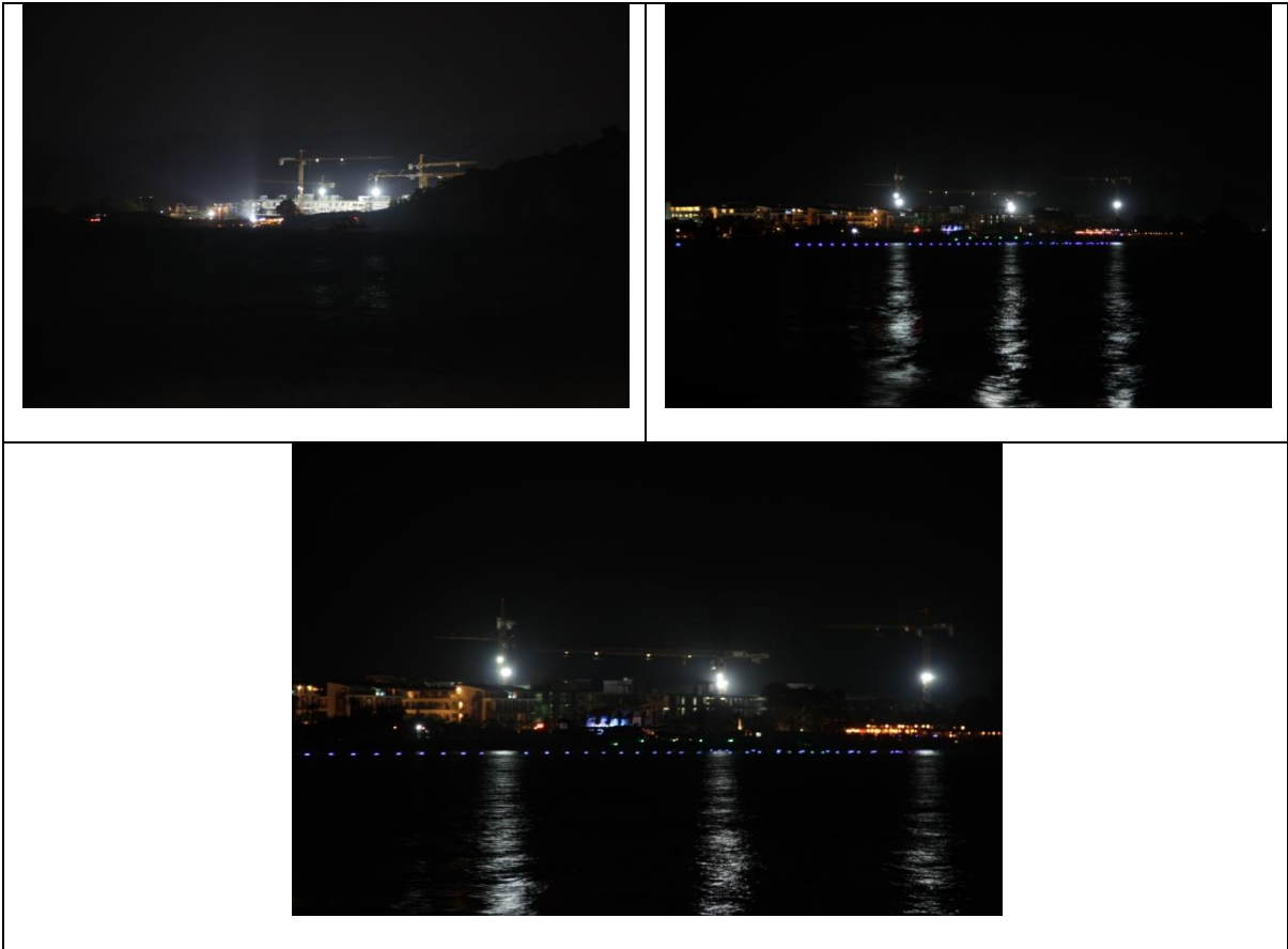
Fig.55. Fethiye SPA. Construction of the new hotel continues at night, and can be seen from every section in the entire SPA. Note the dim blue lights of the quay between the other two hotels in 55b-c.
