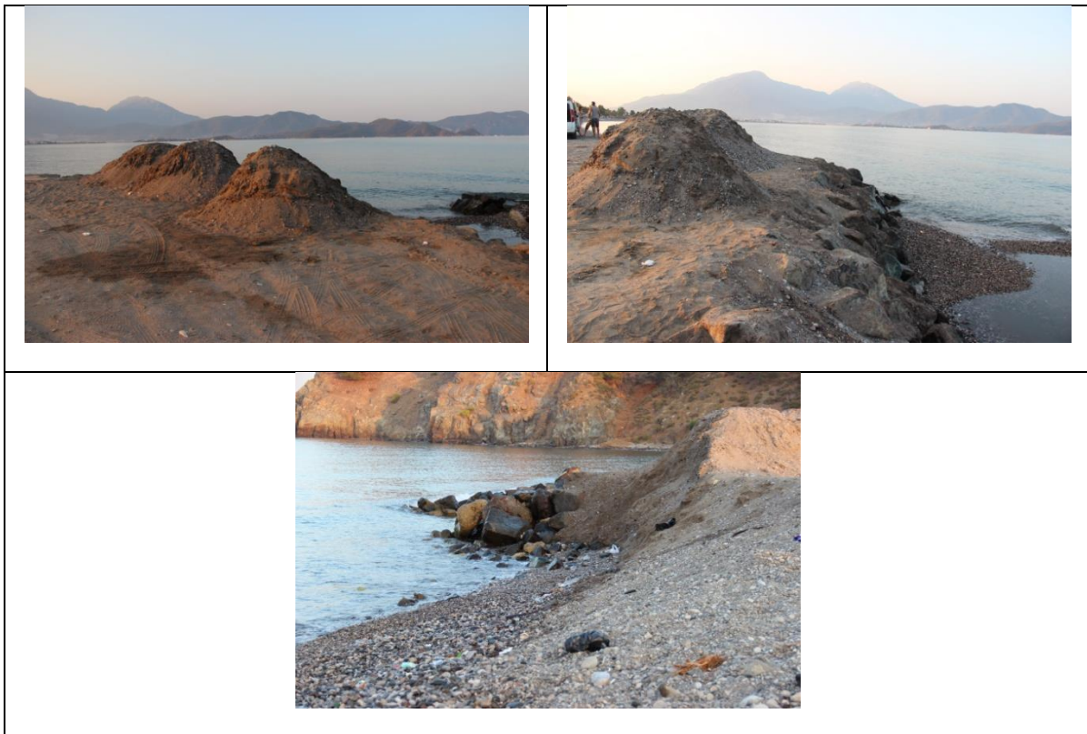
Fig.47. Fethiye SPA, Çalış B. Sand piles near the drainage channel's outlet.
