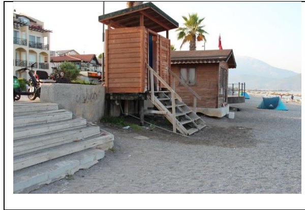
Fig.19. Fethiye SPA, Çalış A. Shower cabins draining directly onto the beach. Note tents further in the background.
