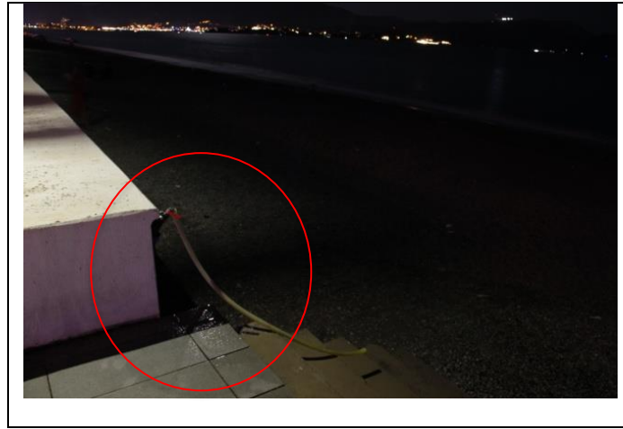
Fig.2. Fethiye SPA, Çalış A. Hose installed at the beach entry point, directly leaking onto the sand.
