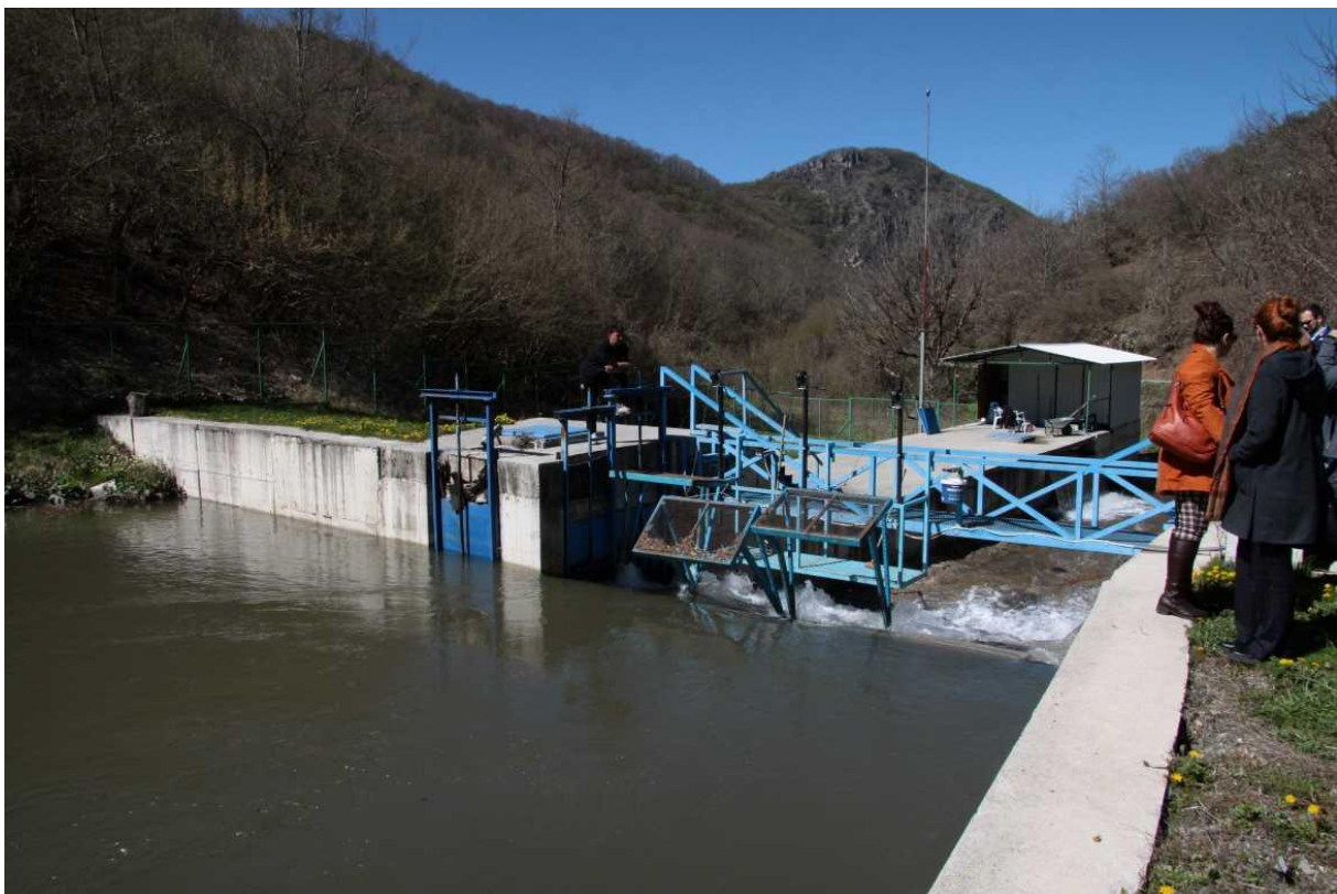
Photo 3: Withdrawal of water for the sHPP – River Recica. @A.Sovinc.
