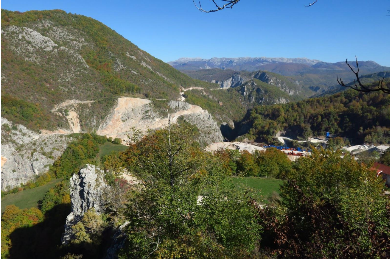
Ongoing construction of Ulog HPP, October 2022
