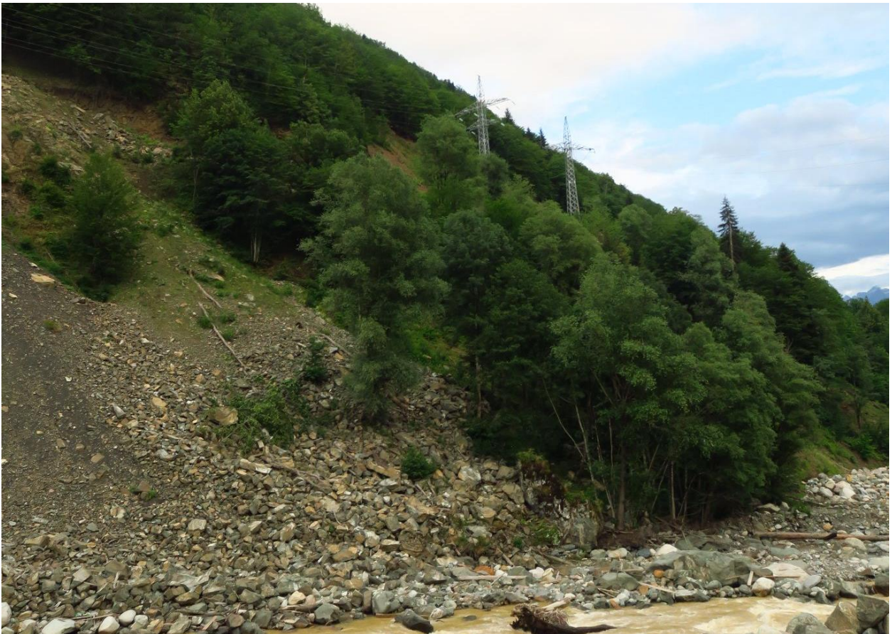
Transmission lines above the river Nenskra, July 2021
