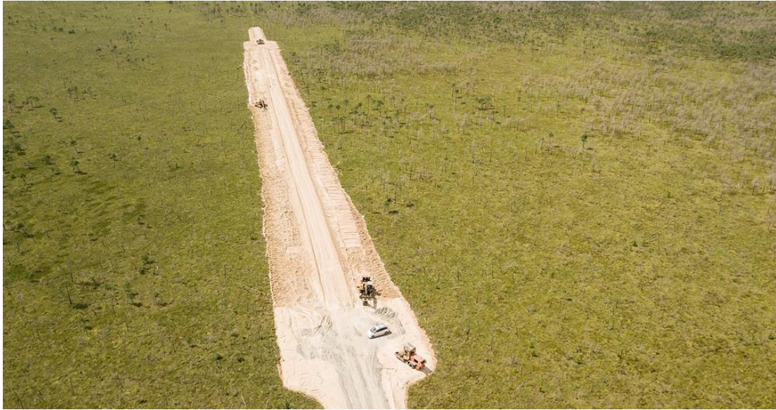
Picture 1. Forest road #3 traversing pristine raise bog during construction.
