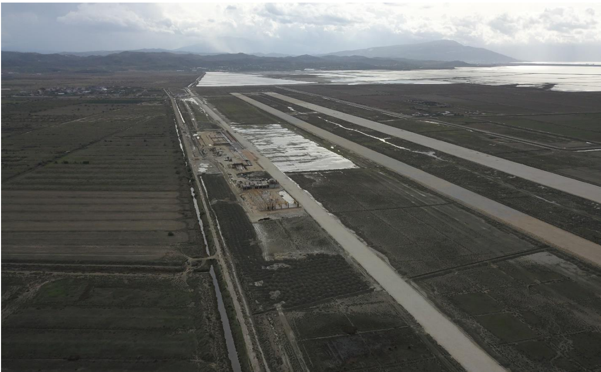
Figure 1: Airport construction site on November 2023 © Arsen Roshi
