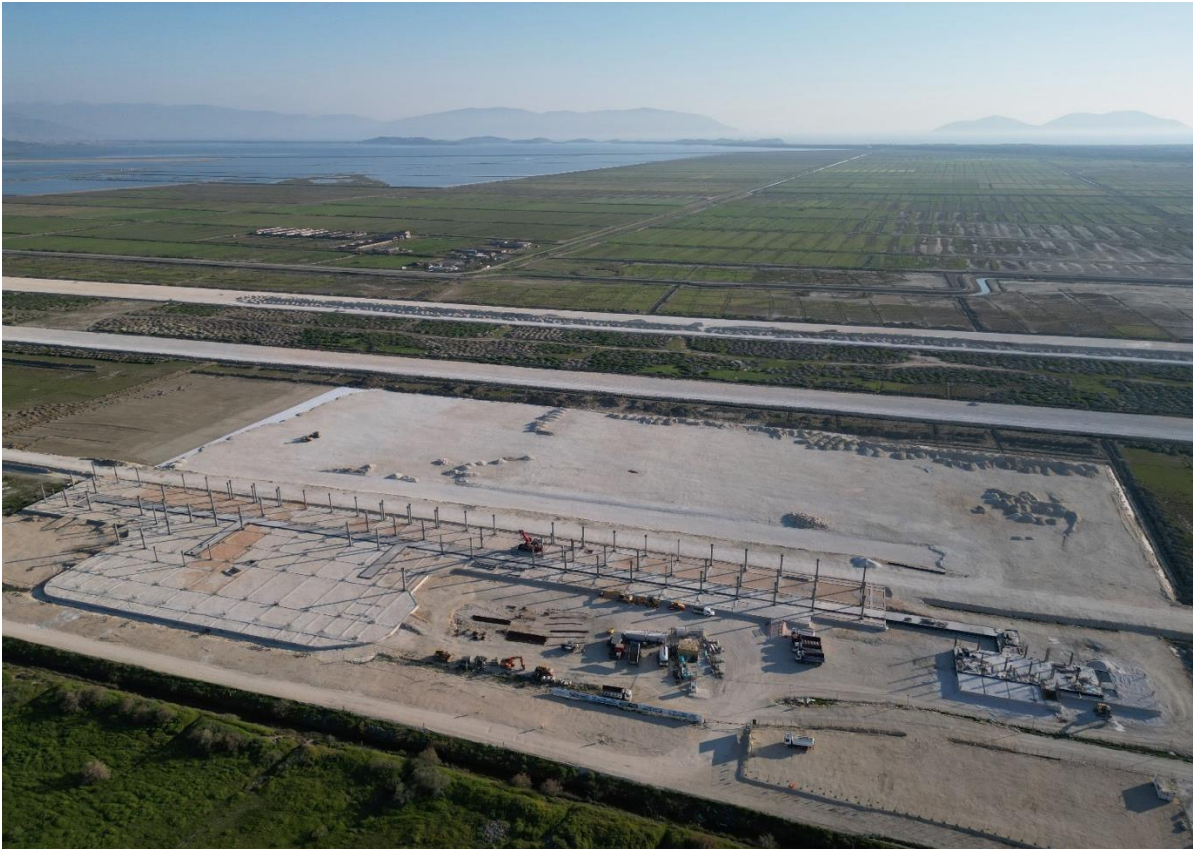
Figure 2: Airport construction site on April 2024 © Arsen Roshi
