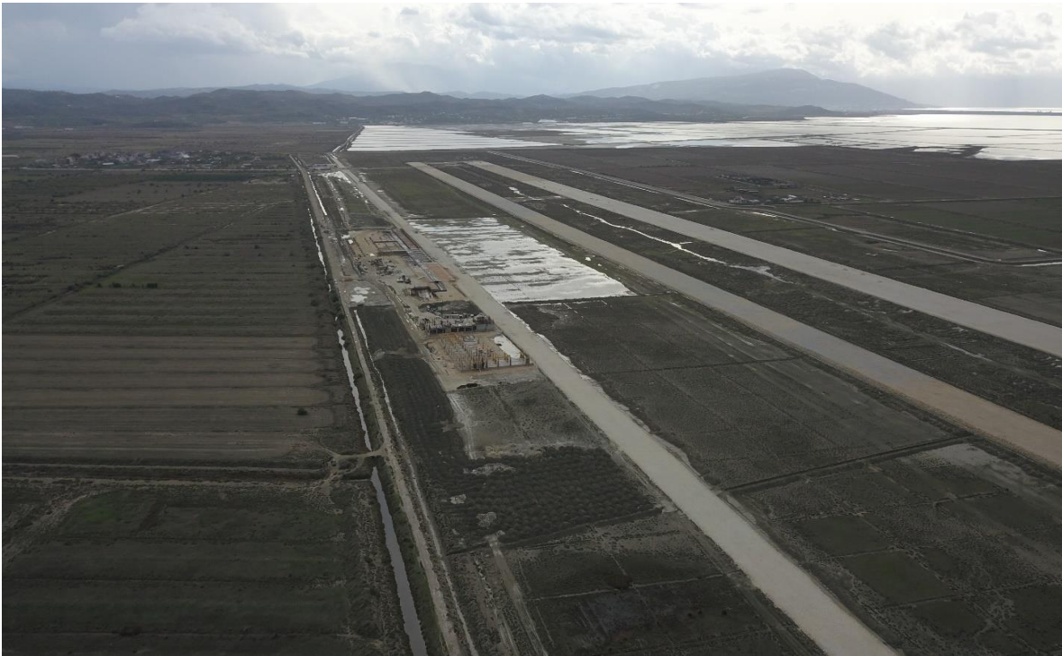
Figure 1: Airport construction site on November 2023 © Arsen Roshi
