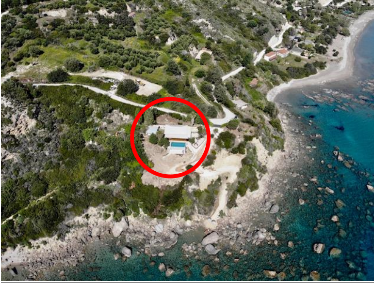
Fig. 2 Illegal building, continuous illegal constructions at the surrounding area
