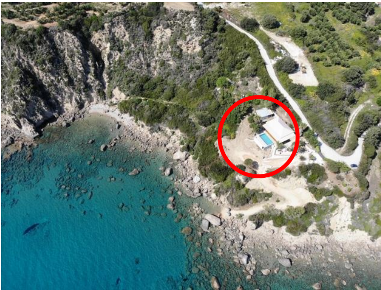
Fig. 3 Illegal building, continuous illegal constructions at the surrounding area
