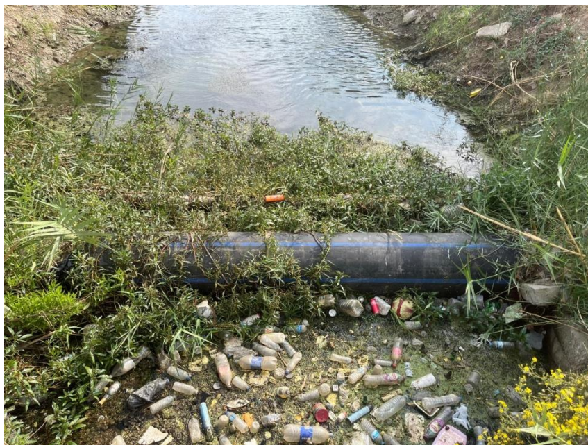
Fig. 14 c) Pollution in the stream next to Anamur 82 facilities
