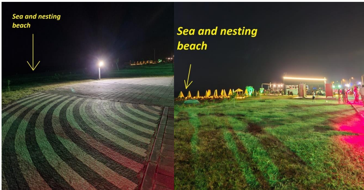
Fig. 13) Lighting poles at the bottom of the beach area where sea and turtle nests are located in Devlet Bahçeli Park. September 2024
