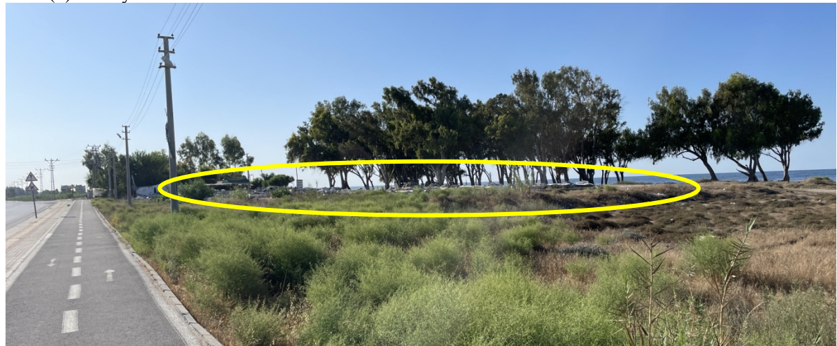
Figure 16. The demolished wedding hall and the remaining rubble (yellow ellipse).
