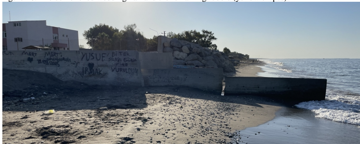
Figure 17. The concrete canal next to the school and the barriers protecting the school from waves.
