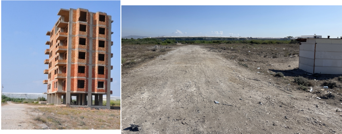
Figure 15. The abandoned building has been completely demolished and the debris cleared away (a) in 2023 (b) in July 2025
