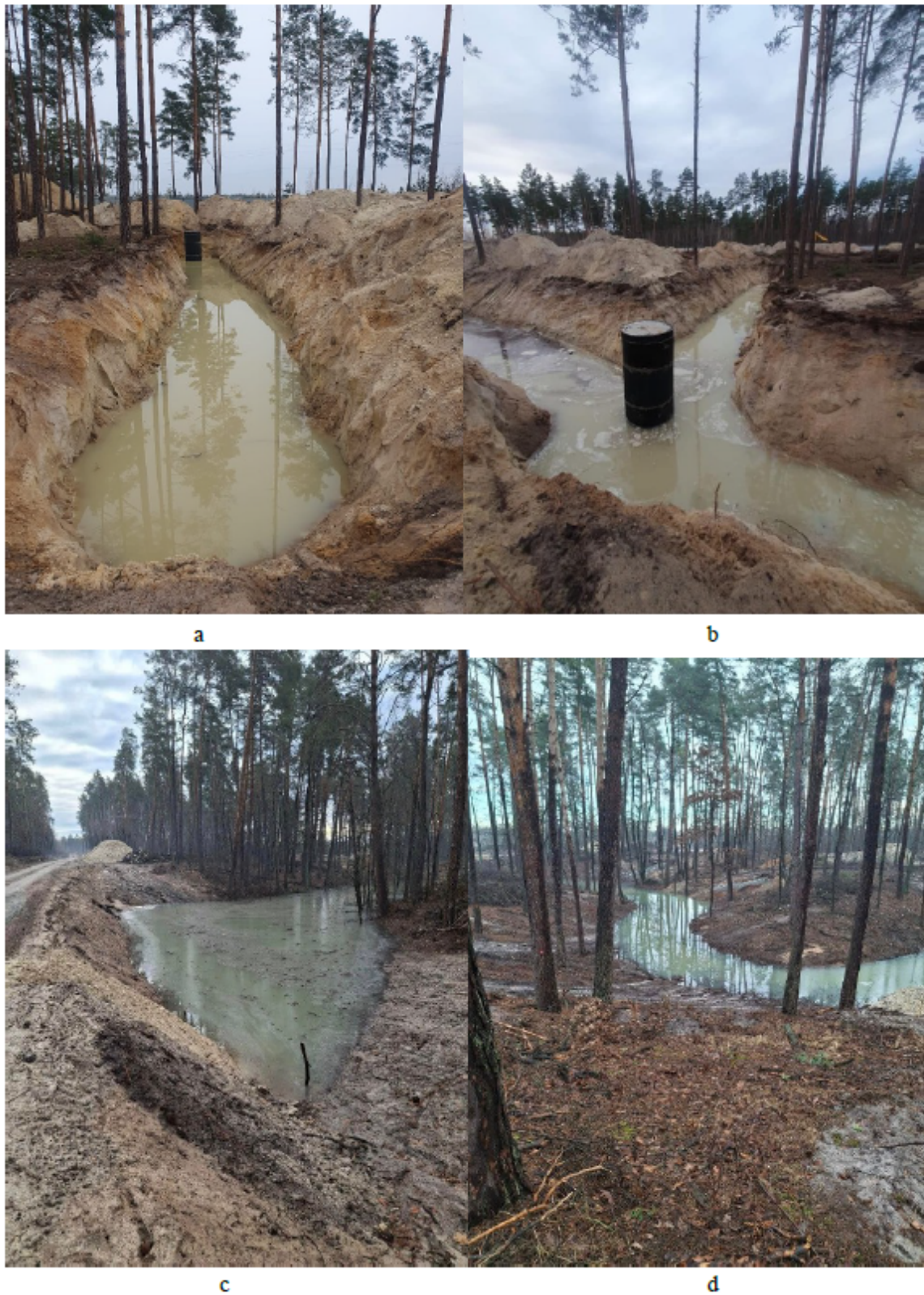
Fig. 17. Natural water level within the NMMC on December 22, 2024, and the installation of a drainage system to support cemetery construction (a, b); works carried out to block the river channel without installing a culvert (c, d).
