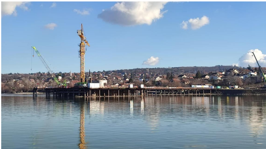
Photo 1 Construction of the main bridge followed by auxiliary bridge
