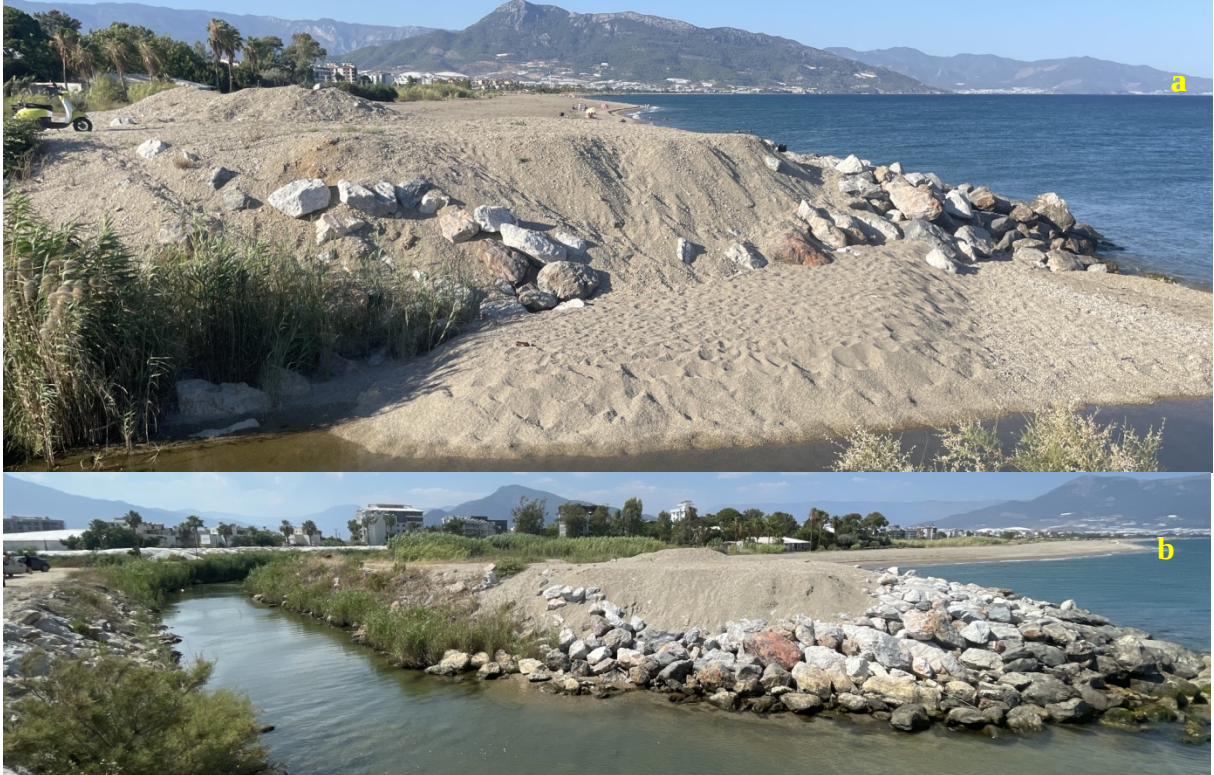
Rock-filling activities carried out in the coastal area where beach formation had begun: July 2025 (a) and June 2026 (b).
