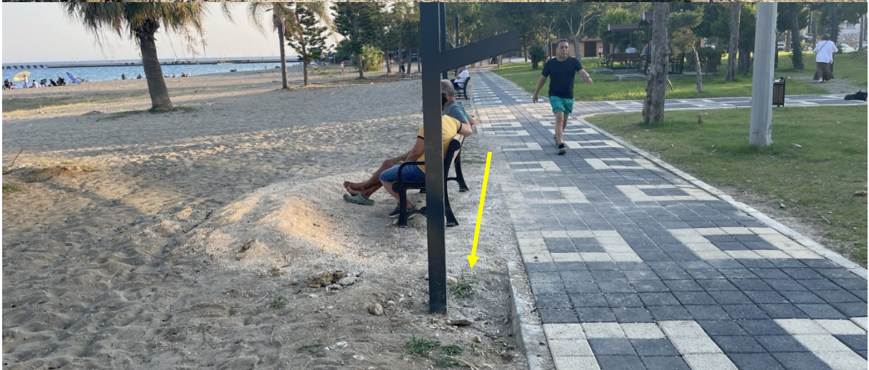
Electrical wiring installed in July 2025 to illuminate the park's walking path, and the subsequent park lighting fixtures installed in June 2026 (area marked in yellow).
