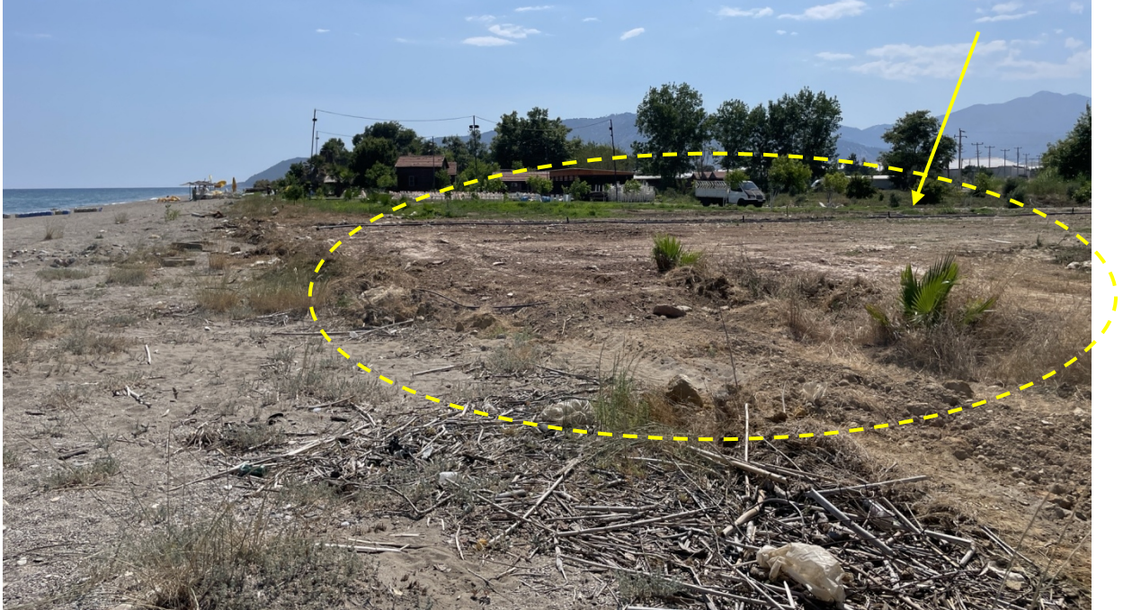
Karaağaç, June 2026: Fertile soil was brought in for saplings, and an irrigation system was installed.
