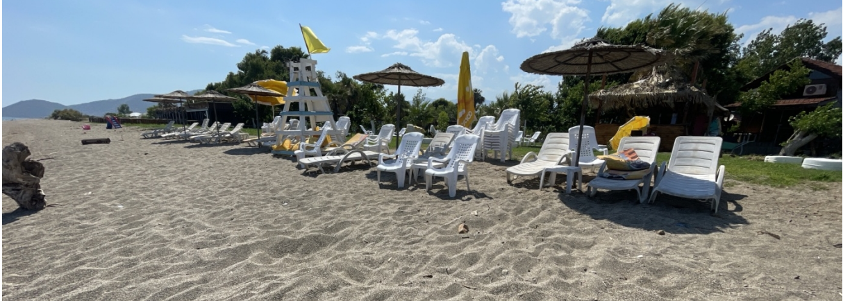
The construction of a new restaurant building and ongoing installation works of new pavilions on Karaağaç Beach by the local bungalow enterprise.
