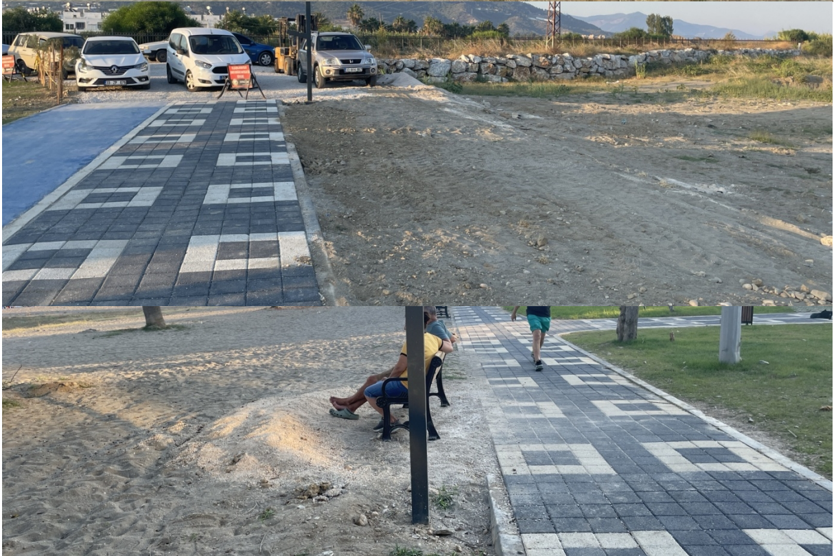
The setback/relocation of the walking path further inland at Rauf Denktaş Park: May 2025 (a) and June 2026 (b).
