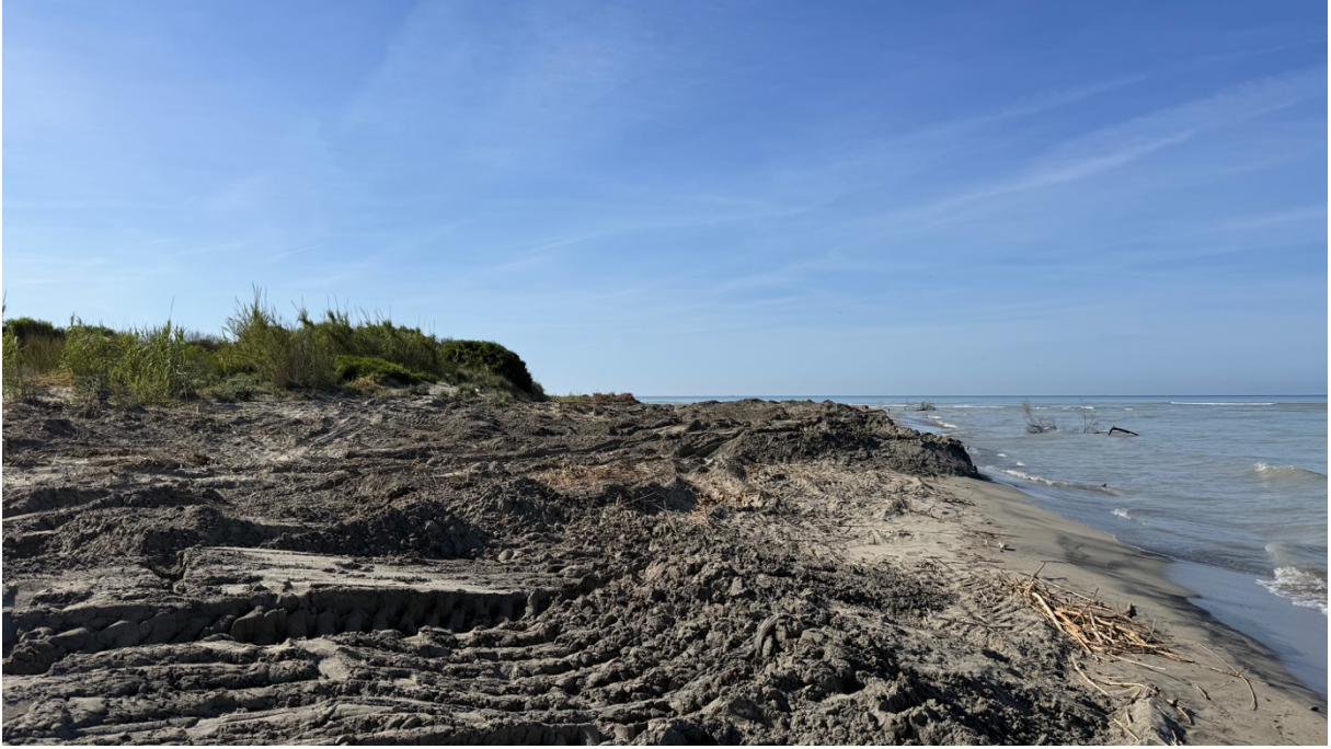
A temporary dune barrier system was constructed to prevent vehicle Access at the mouth of Eşen River.
