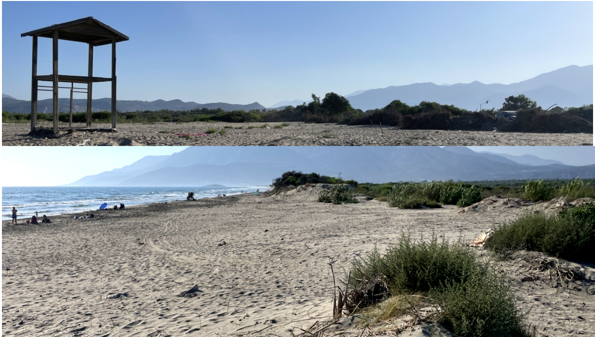
The status of abandoned wooden structures disrupting beach integrity on Letoon Beach in 2025 (top), and the current state of the site in 2026 showing their complete removal and clearance (bottom).
