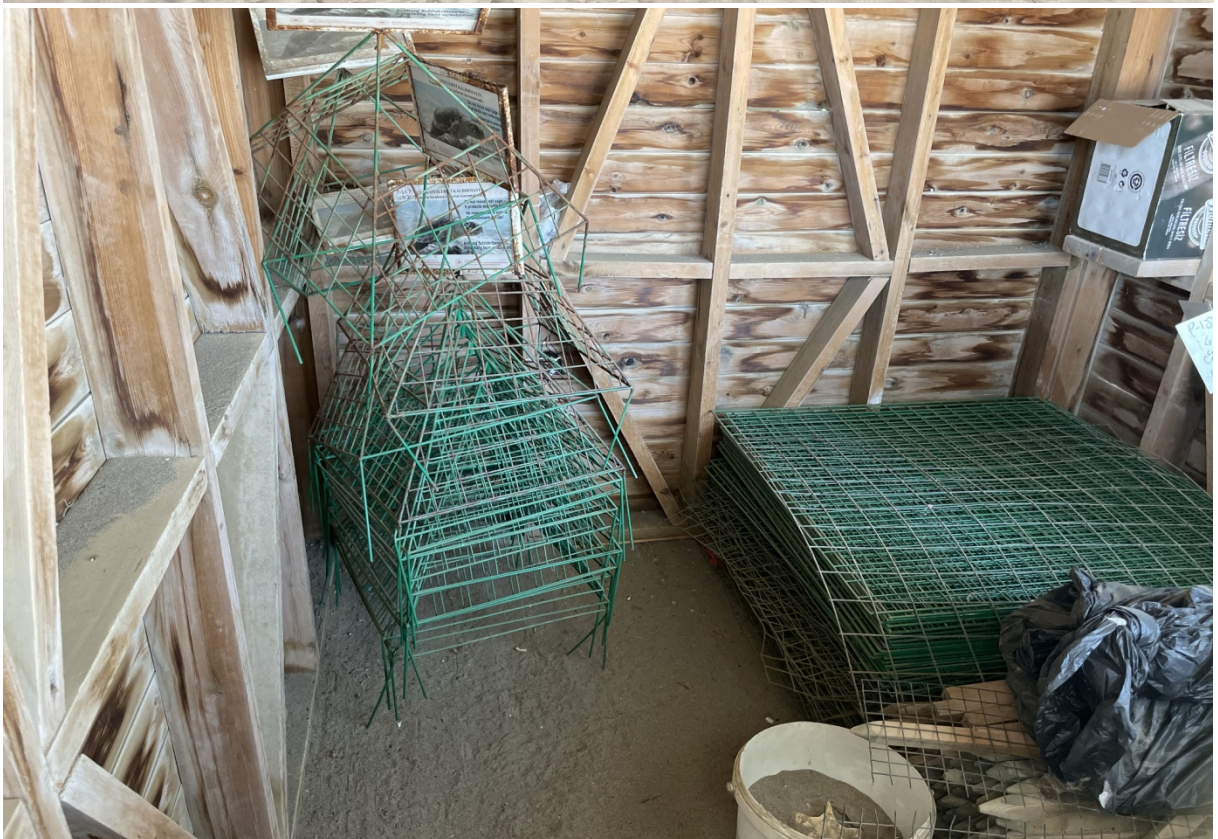
Information kiosk; used more as a cage storage than for providing information.
