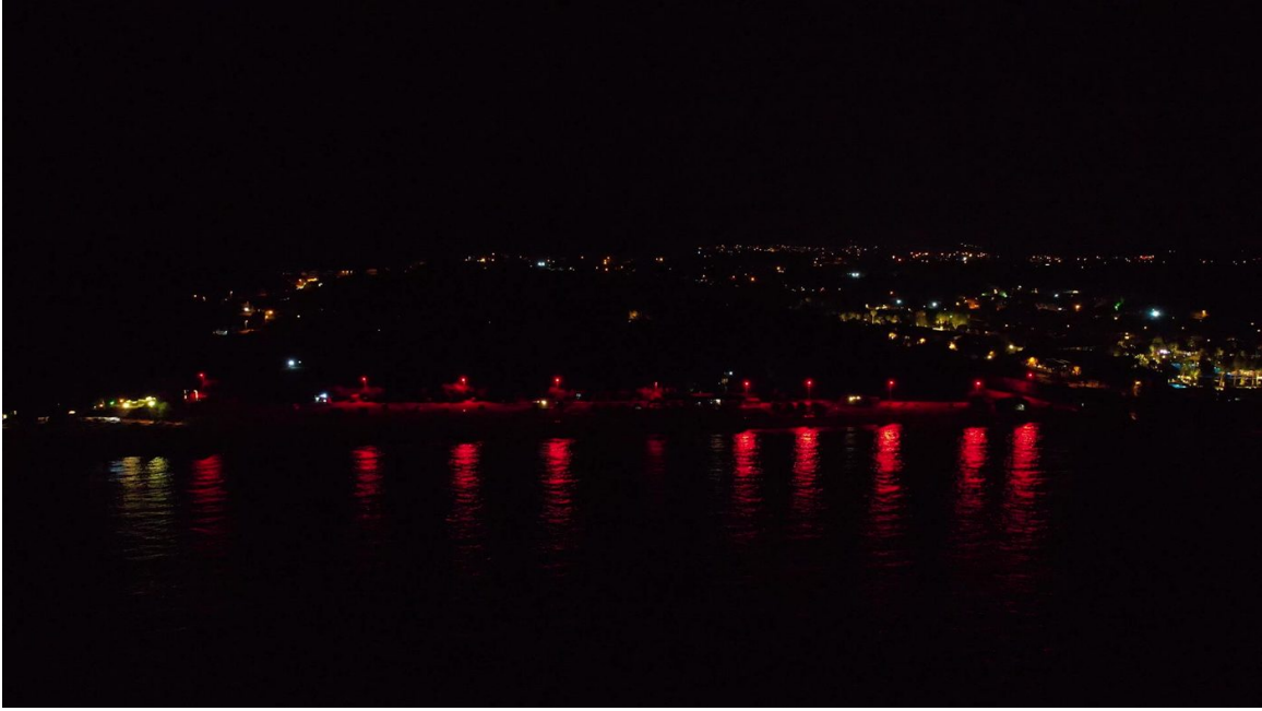
Red street lighting installed along the coastline (Fig. 17)
