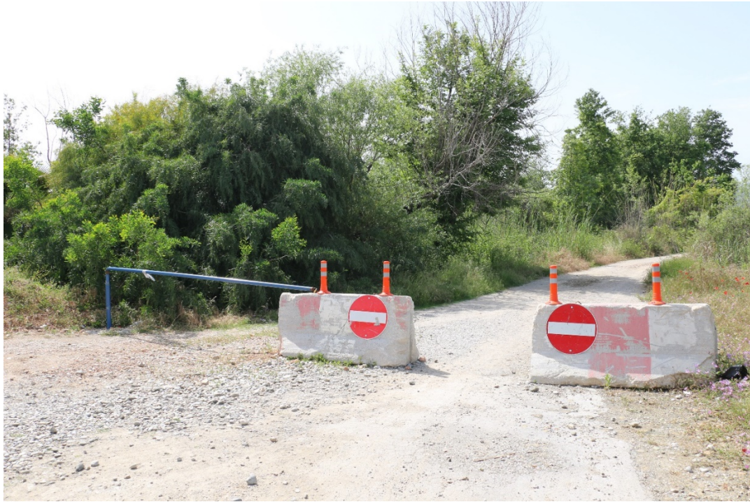
Karaot Beach closed off with concrete barriers (Fig. 11)
