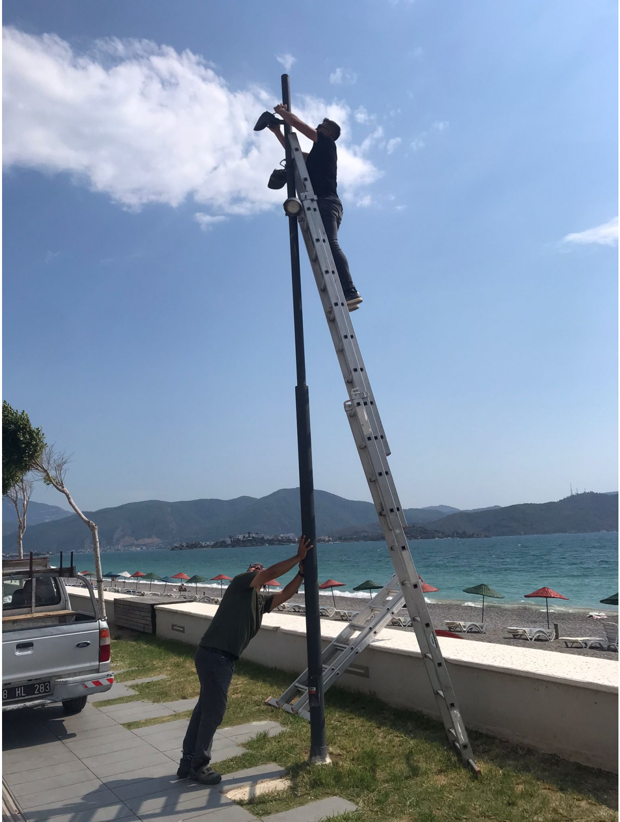
Correction work in the area (Fig. 10)
